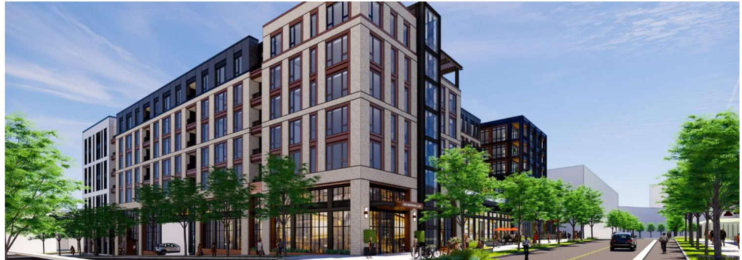
Northeast corner at Westend Blvd/Road 1 and Verve St/Road 5
