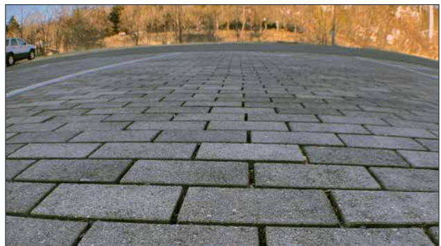
Permeable pavement
