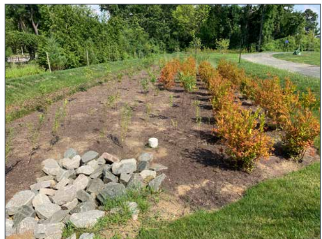
Bioretention facility
