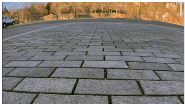
Permeable pavement
