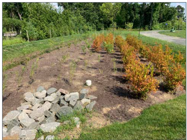
Bioretention facility
