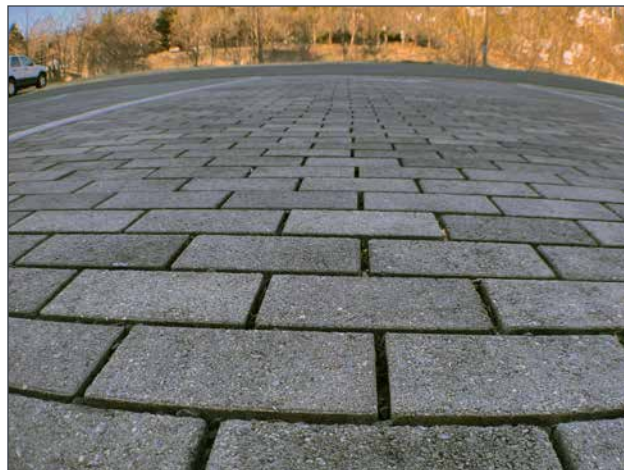
Permeable pavement
