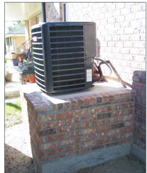
Elevated exterior HVAC equipment SOURCE: FEMA
