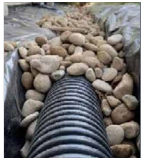
French drain around basement SOURCE: CITY OF ALEXANDRIA
