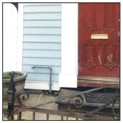
Meter may be placed on front façade if it is a safety risk to be located in the basement. A pressure relief vent may be located on the front or side façade. Paint all to match adjacent wall color.
