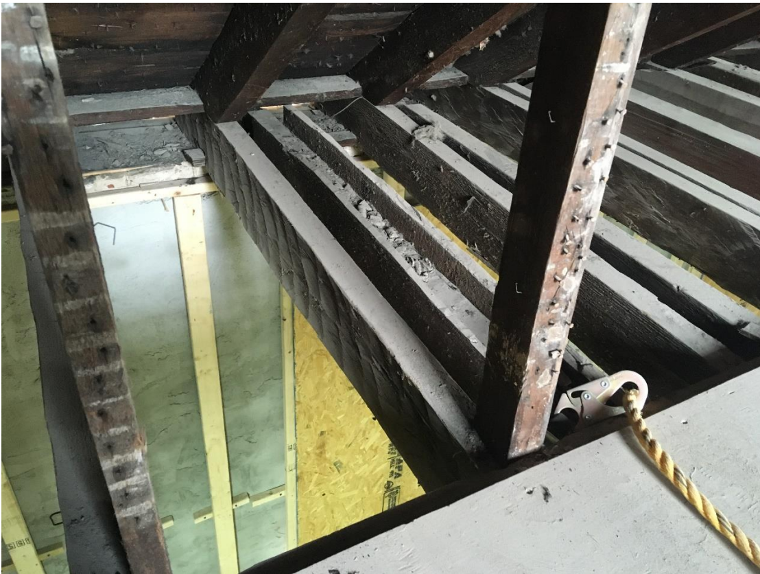
Figure 6: Hewn Ceiling Joists
