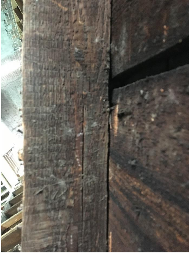
Figure 7: Pitt Saw Marks on the Rafters
