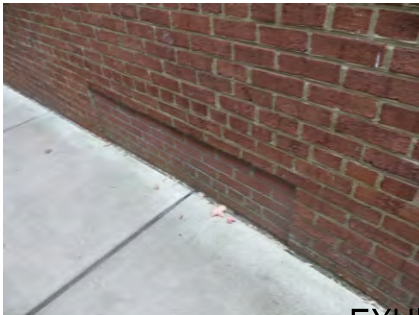
DETAIL-TYPICAL LOWER SIDE WINDOW -BRICKED
