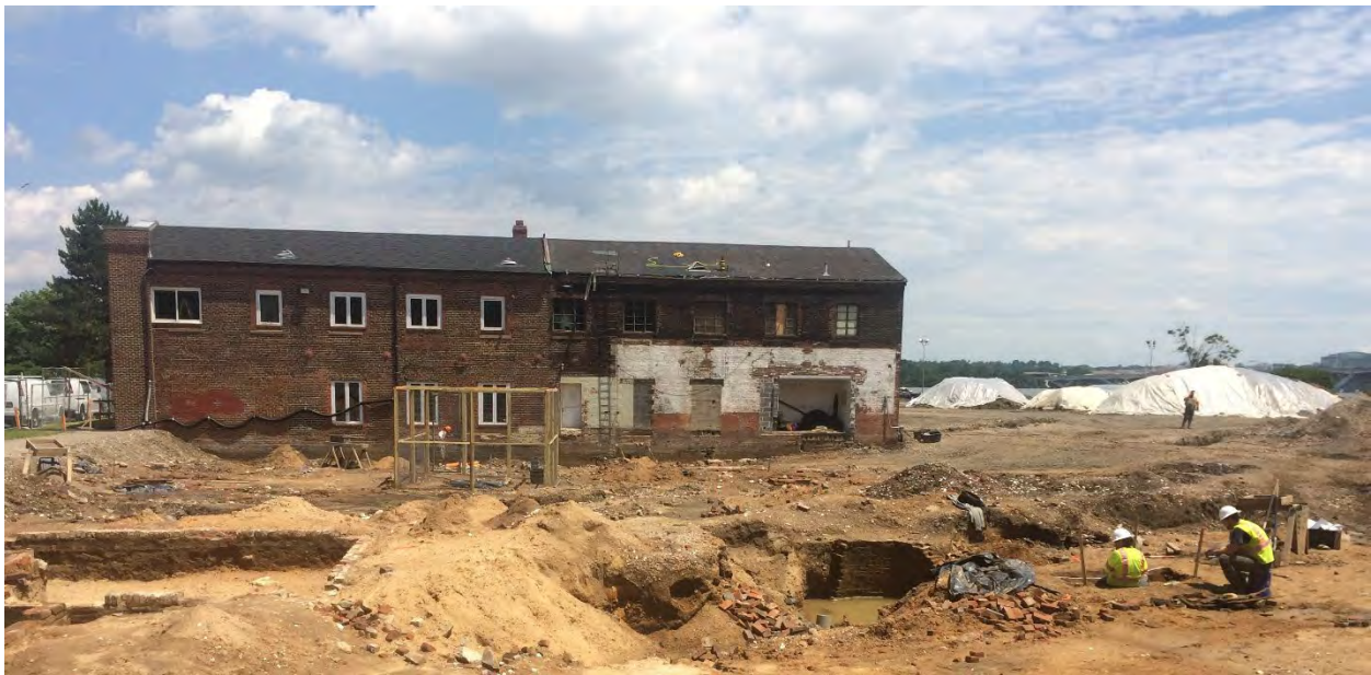
Figure 1: Image of the west elevation of 10 Duke in 2017 showing the variety of existing window types and masonry coatings to be removed.
