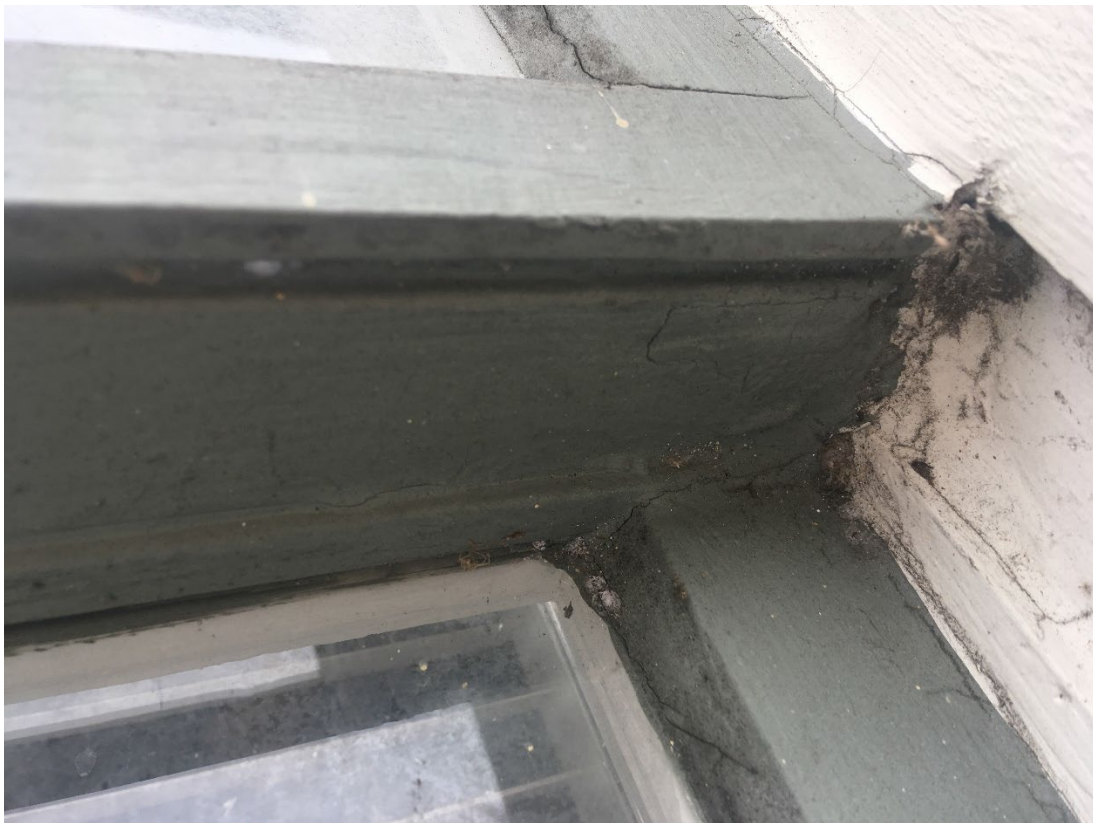
Figure 1: Image showing drip edge routed in the upper sash, typical throughout. This is not a common feature of Victorian period window sash.
