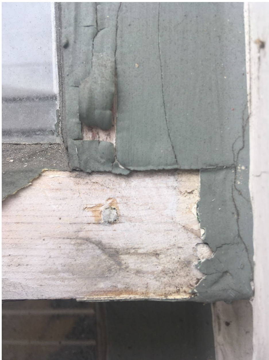
Figure 2: Iron finish nails at stile and rail joint, typ.
