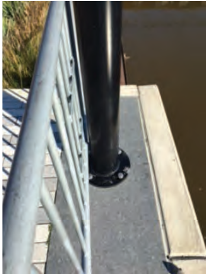
Light post installed in granite band with ~8" concrete reveal
