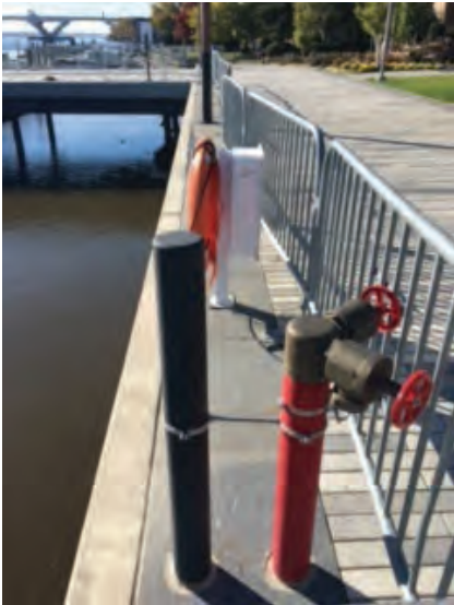
Standpipe/support pipe and Life Safety Station (beyond)
