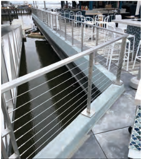
Guardrail installed at northern end of RTS pier
