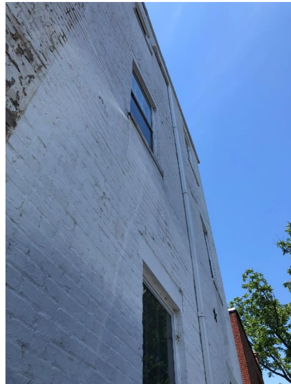
Photo 7: Outward Bowing of East Wall
