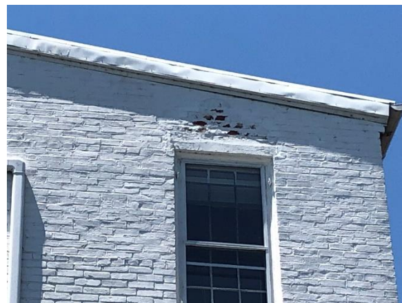
Photo 4: Brick deterioration over lintels
