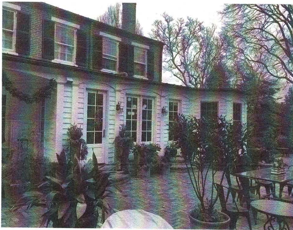
South elevation, octagonal bay to have octagonal cupola on roof porch enclosure (at left) shall have matching siding, pilasters, segmented arches as existing
