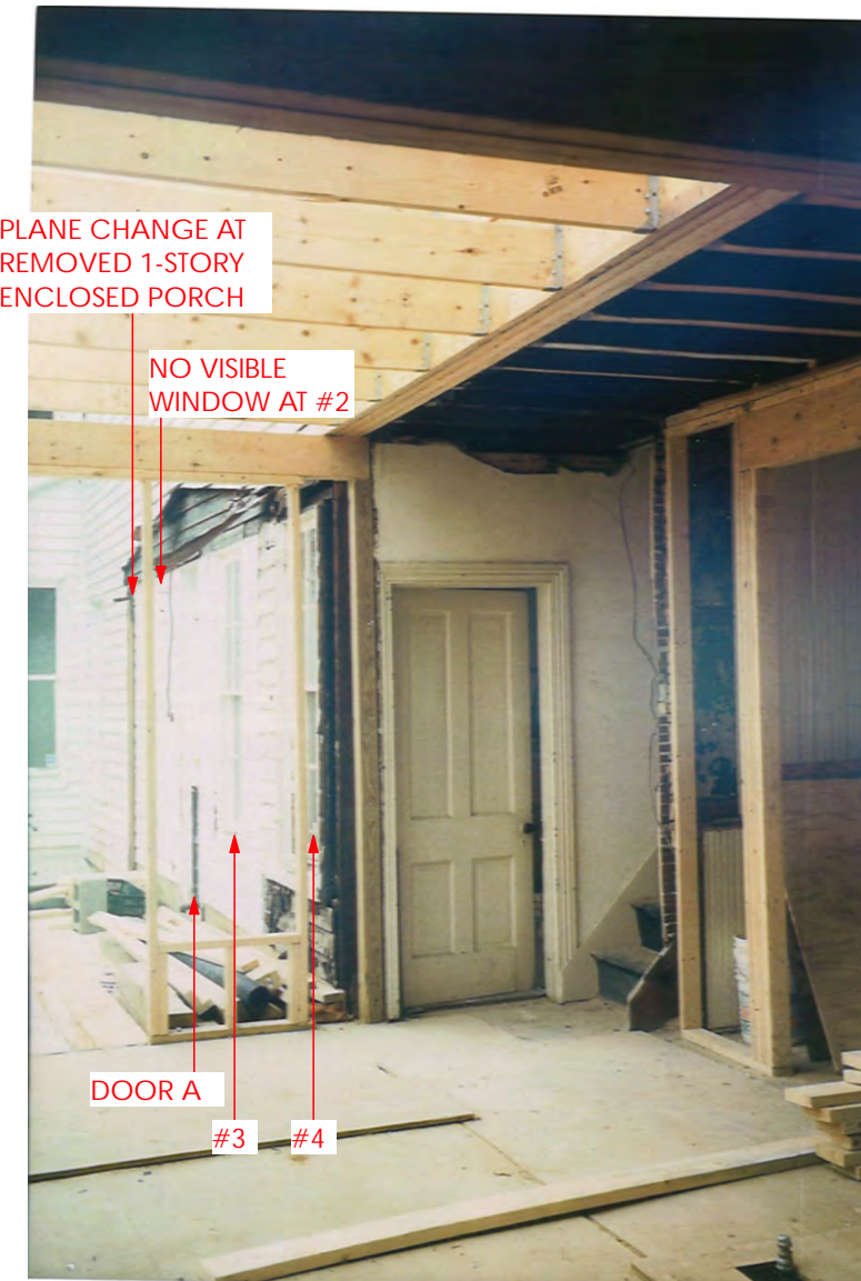
FIRST FLOOR EXISTING CONDITIONS DURING 1999 ADDITION
