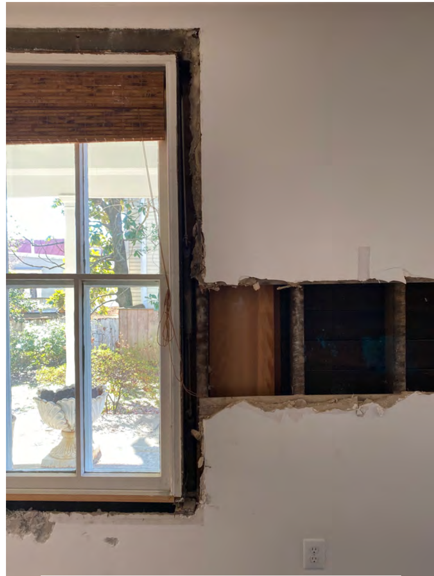
FIRST FLOOR WINDOW #2 - WINDOW FRAME/WEIGHT POCKET IS SHOWN IN NEW FRAMING
