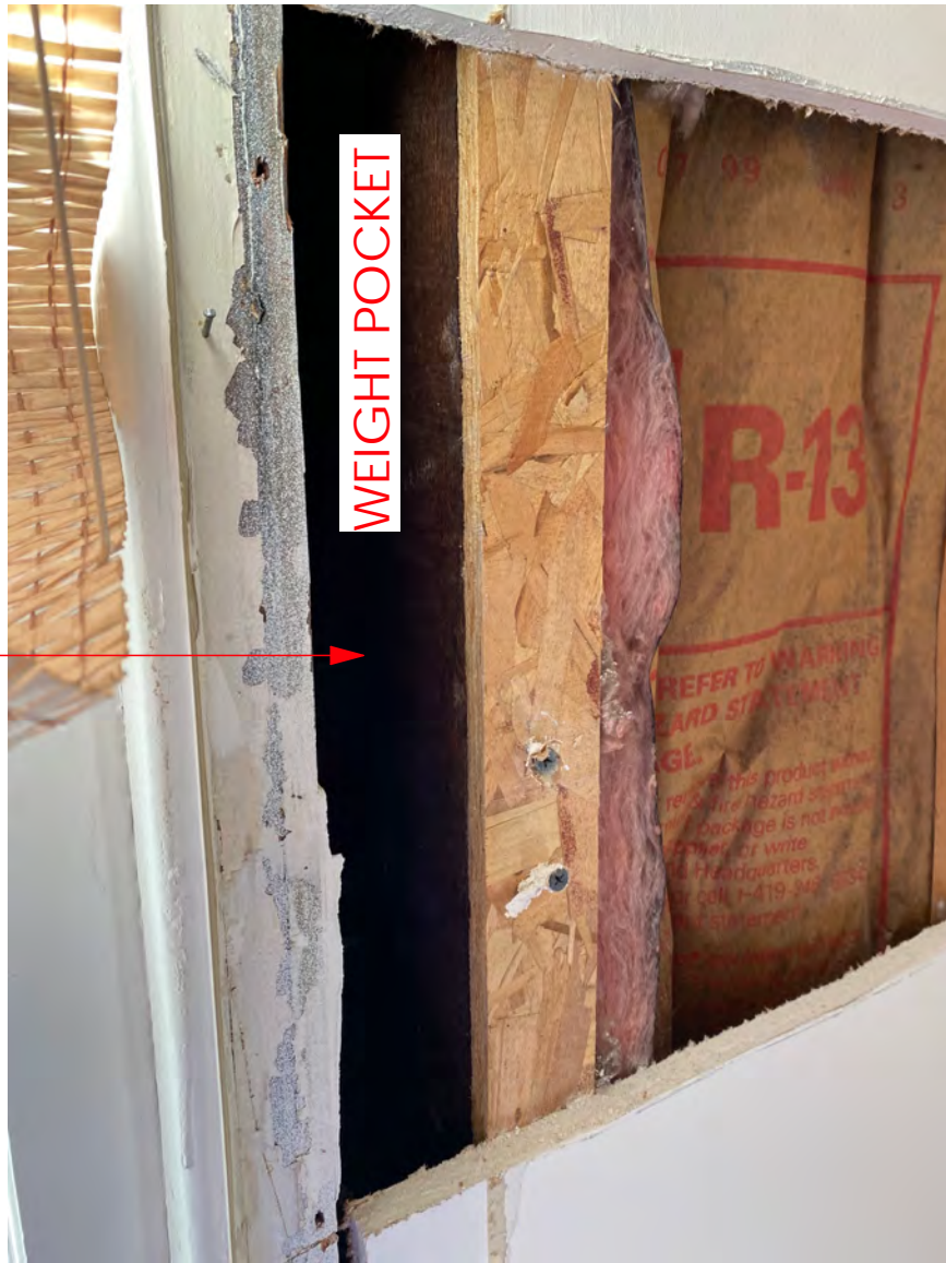
WINDOW #5 APPEARS TO BE AN ORIGINAL OPENING, HOWEVER THE BOTTOM SASH (AND POSSIBLY THE UPPER SASH) IS A NEWER REPLACEMENT. THE CORDS IN THE WEIGHT POCKET ARE NEWER, AND THERE ARE TWO WEIGHTS IN THE POCKET
