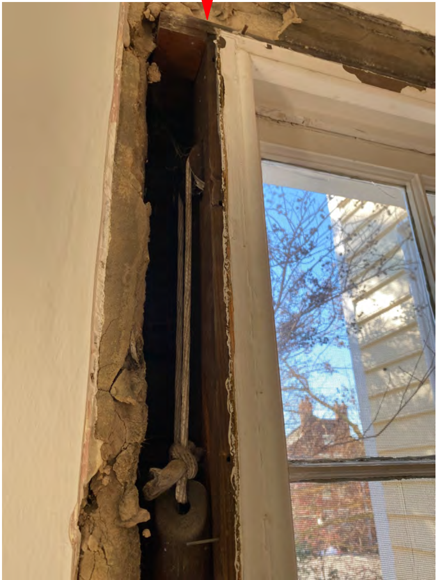
SECOND FLOOR WINDOW #1 SHOWS AN APPARENT ORIGINAL OPENING; THE NOTCHED HEADER INDICATES A POSSIBLE REPLACEMENT WINDOW AT SOME POINT IN TIME
