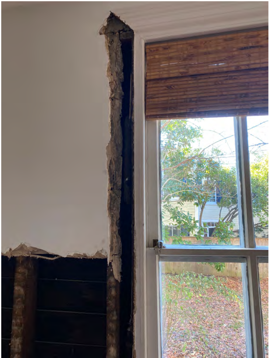
FIRST FLOOR WINDOW #1 SHOWS AN APPARENT ORIGINAL OPENING
