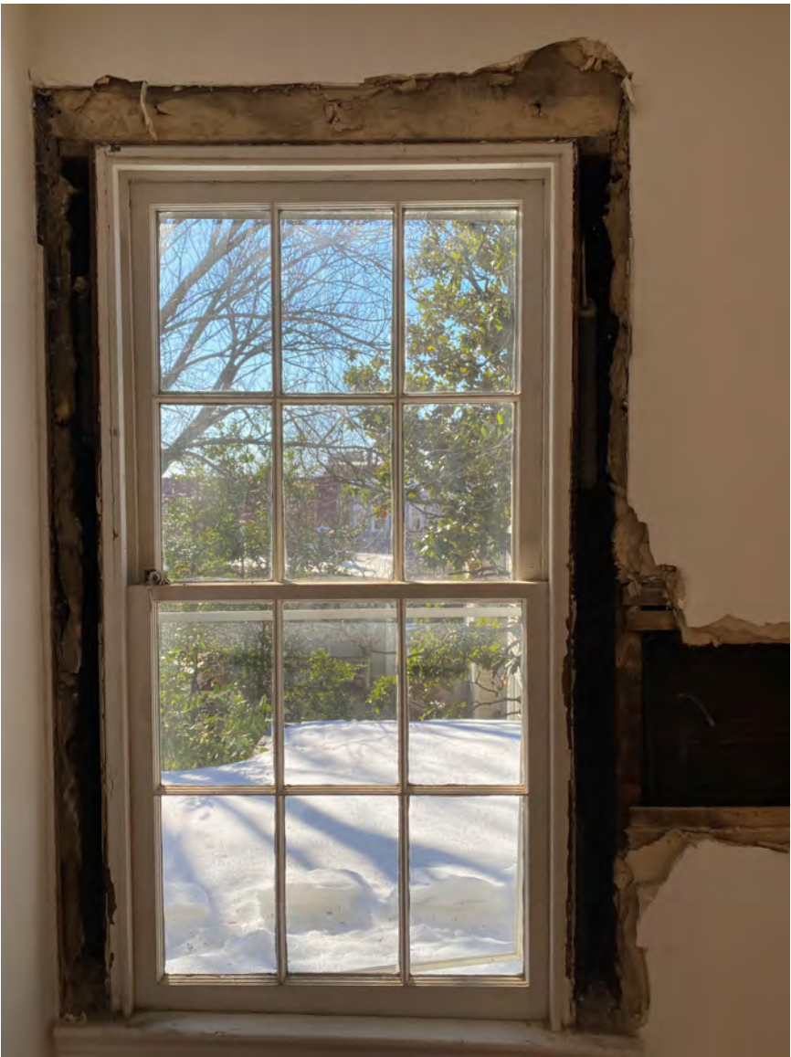
WINDOW #4 APPEARS TO BE AN ORIGINAL OPENING, HOWEVER THE BOTTOM SASH (AND POSSIBLY THE UPPER SASH) IS A NEWER REPLACEMENT. THE CORDS IN THE WEIGHT POCKET ARE NEWER, AND THERE ARE TWO WEIGHTS IN THE POCKET
