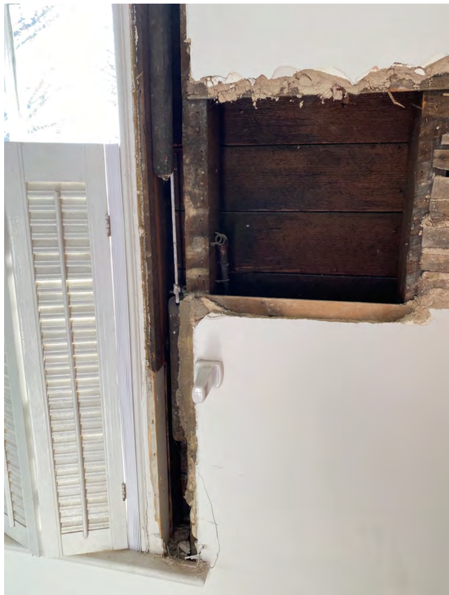
SECOND FLOOR WINDOW #2 SHOWS AN APPARENT ORIGINAL OPENING
