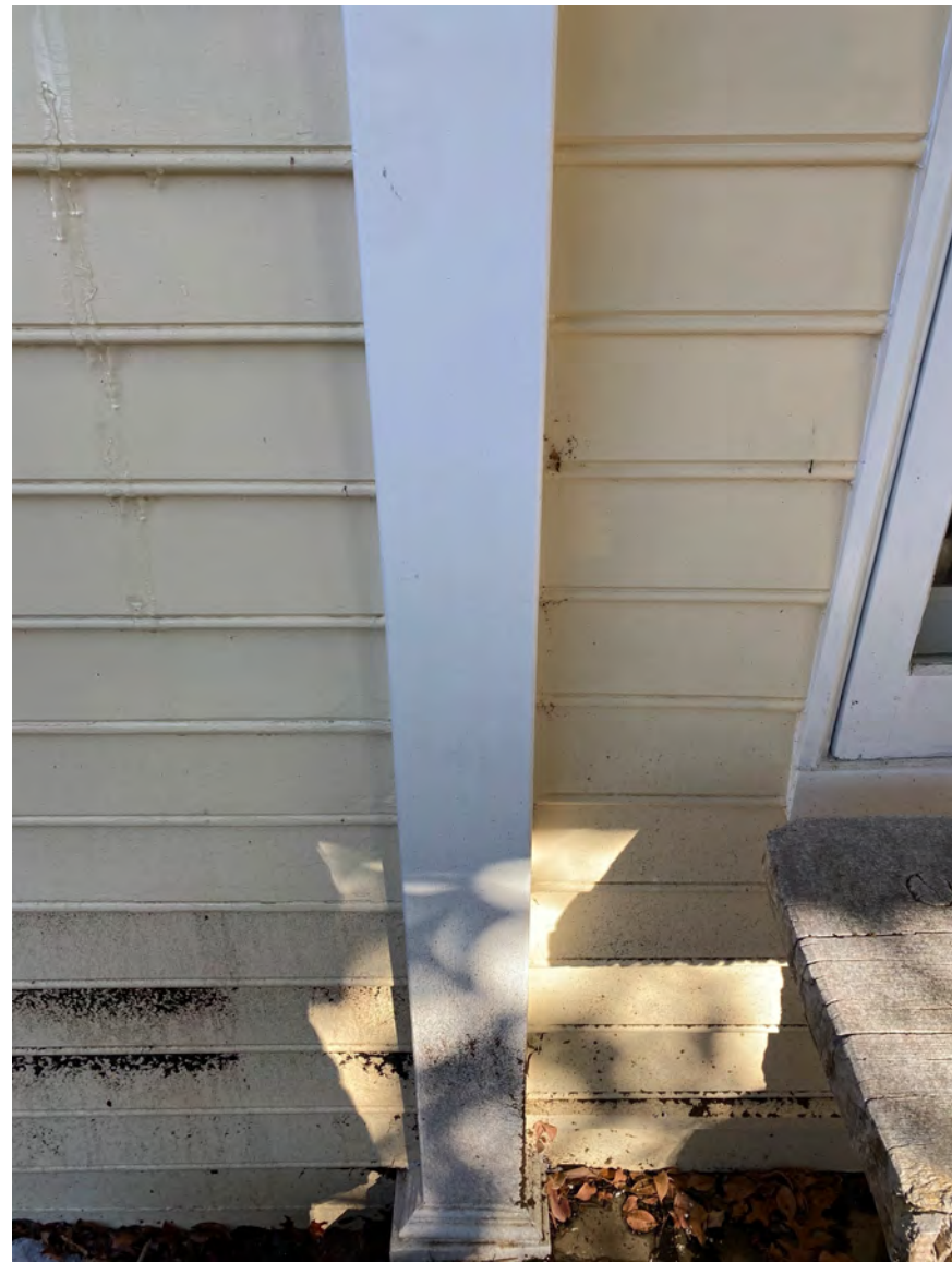
FIRST FLOOR WINDOW #2 IS SHOWN ON THE EXTERIOR TO THE RIGHT OF THIS PILASTER. THERE IS A PLANE CHANGE IN THE SIDING. THIS IS WHERE THE NEW FRAMING/SHEATHING IS VISIBLE FROM THE INTERIOR
