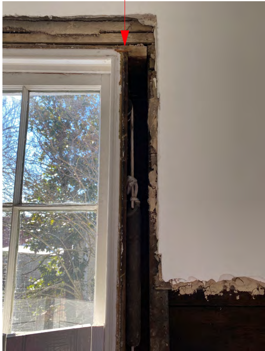
SECOND FLOOR WINDOW #2 SHOWS AN APPARENT ORIGINAL OPENING; THE NOTCHED HEADER INDICATES A POSSIBLE REPLACEMENT WINDOW AT SOME POINT IN TIME
