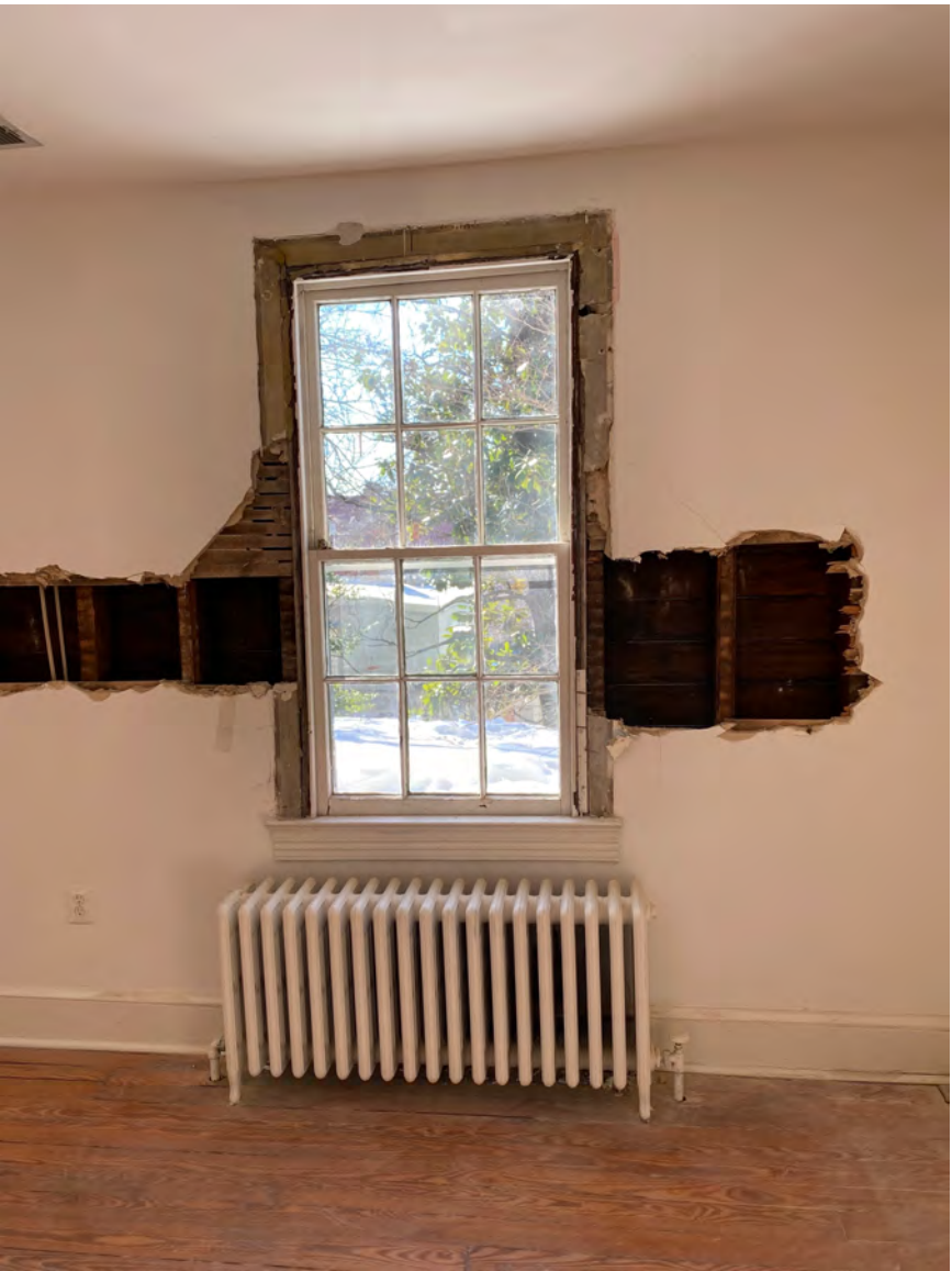
WINDOW #3 APPEARS TO NOT BE ORIGINAL OR AN ORIGINAL OPENING AS THERE IS NO EVIDENCE OF A WEIGHT POCKET LIKE IN THE OTHER WINDOWS ON THE "ELL"
