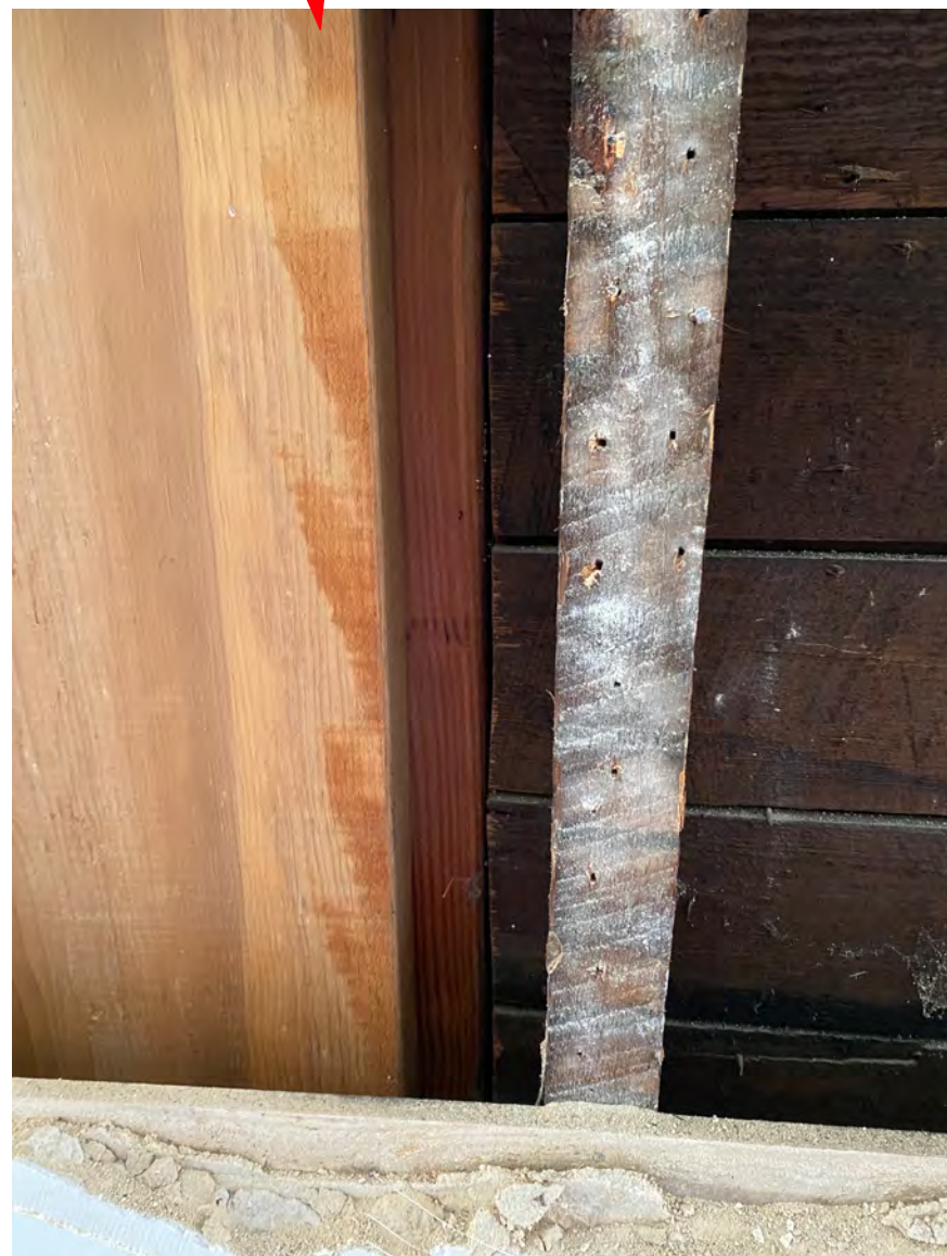
TO THE RIGHT OF FIRST FLOOR WINDOW #2 - ORIGINAL SHEATHING IS CUT ALL THE WAY TO THE FLOOR AND NEW FRAMING/SHEATHING BEGINS; NEW PLASTER IS EVIDENT
