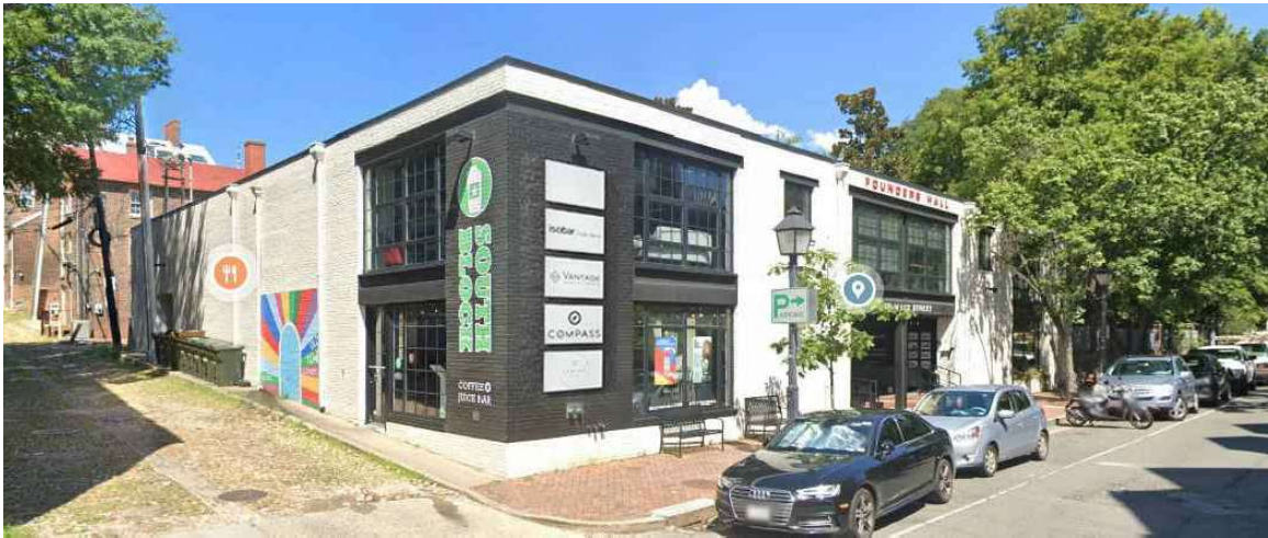
1 EXISTING – SOUTH-EAST CORNER OVERVIEW
