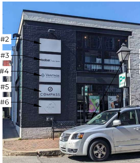
3 EXISTING – EAST FACADE – SIGN #2-#8
