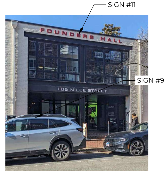
4 EXISTING – EAST FACADE – SIGN #11
