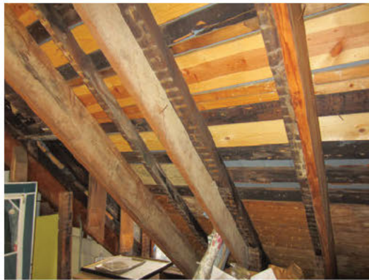
5 PHOTO: EXISTING ATTIC FRAMING A1 NO SCALE
