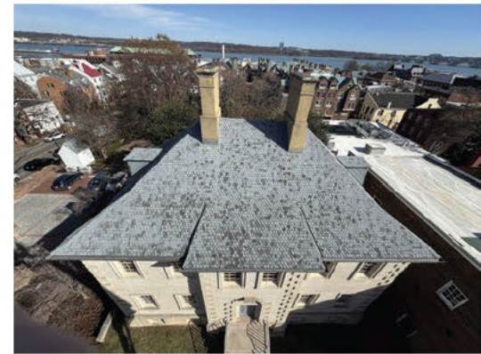
6 PHOTO: ROOF A1 NO SCALE
