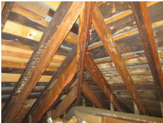
4 PHOTO: EXISTING ATTIC FRAMING A1 NO SCALE
