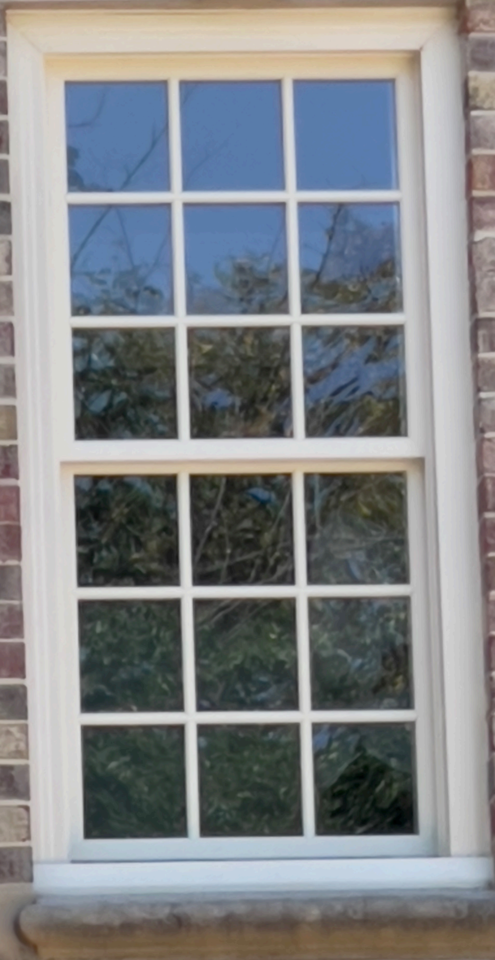
Example of “insert” type Marvin replacement window at 222 Oronoco Street, Alexandria
