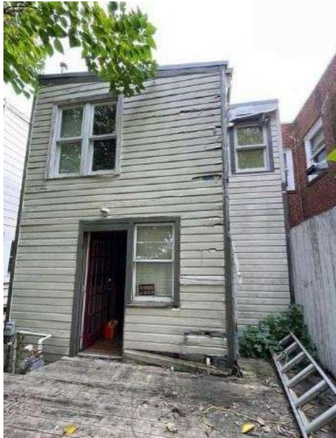
Figure 1: Photo of existing rear elevation.
