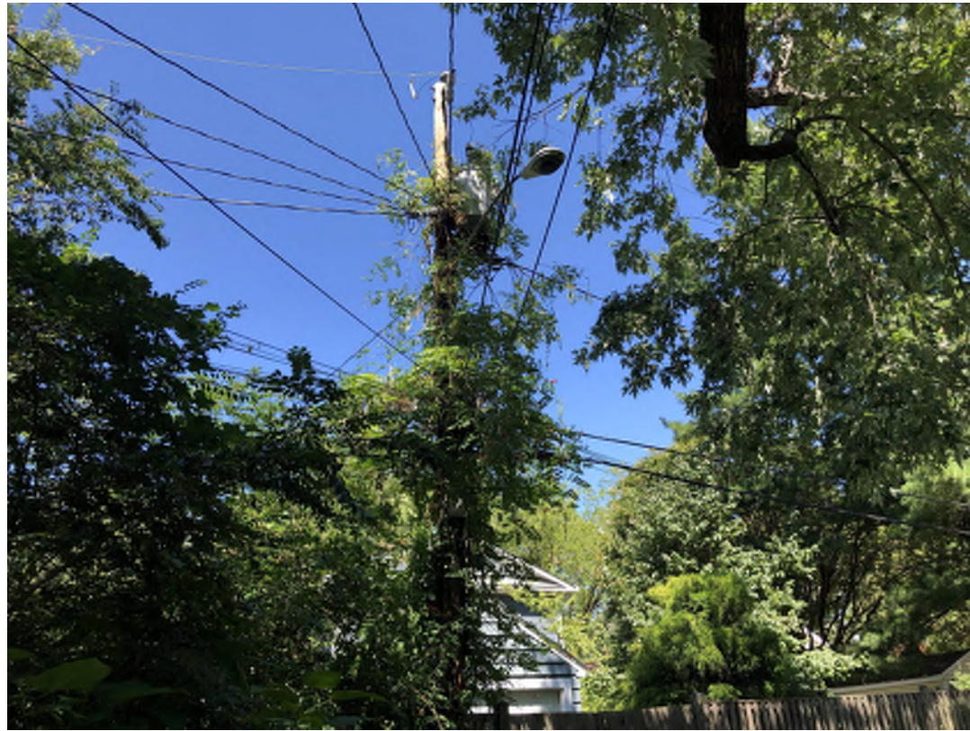
1. EXISTING UTILITY POLE FOR HOMES AT 1405 TO 1411 MT. VERNON AVE. & 404 TO 406 E. ALEXANDRIA AVE.
