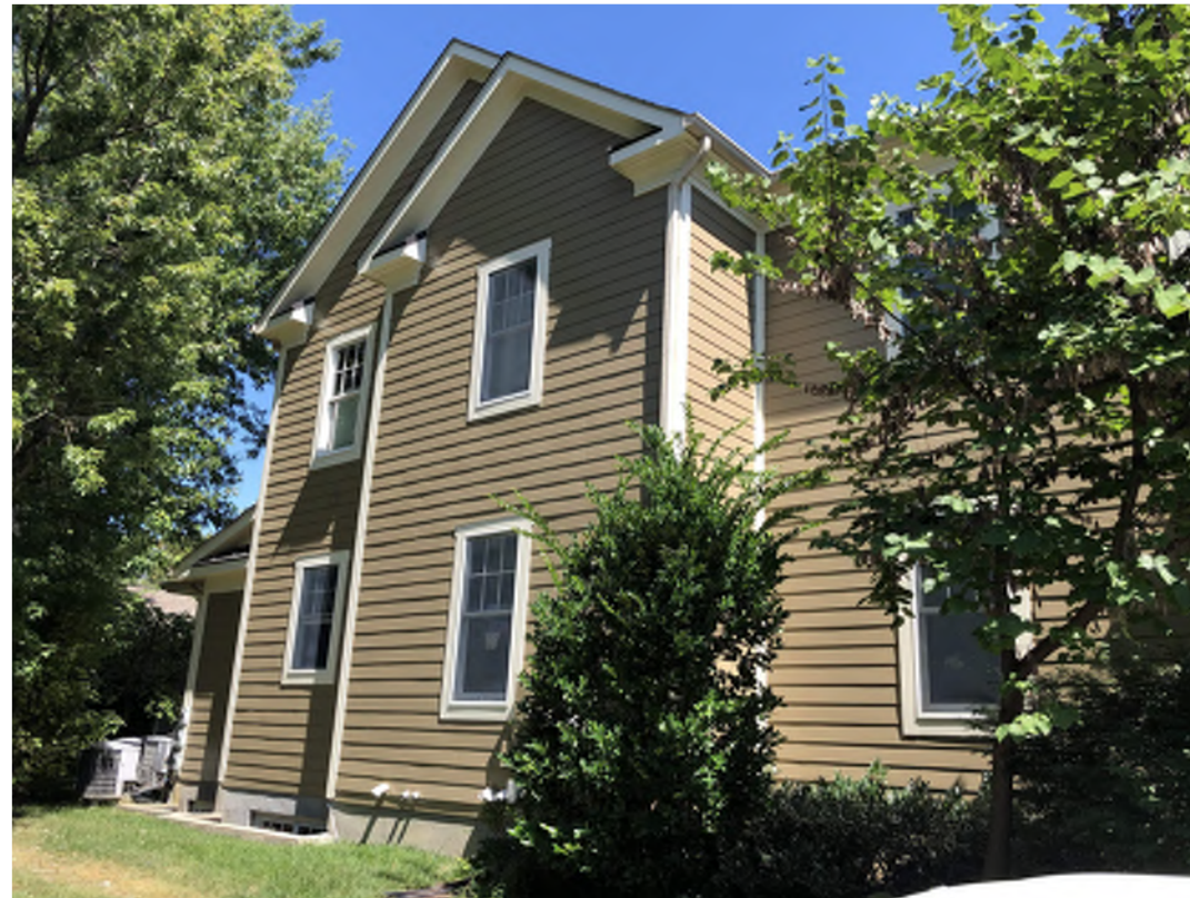
4. 408 E. ALEXANDRIA AVE. WEST SIDE YARD
