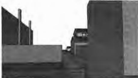
West Facade (side)
