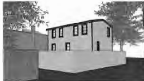
South Facade (rear)
