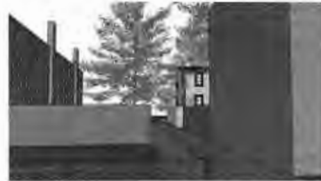
West Facade (side)
