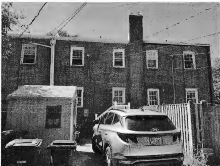
3. REAR FACADES AND YARDS OF 1407 - 1411
