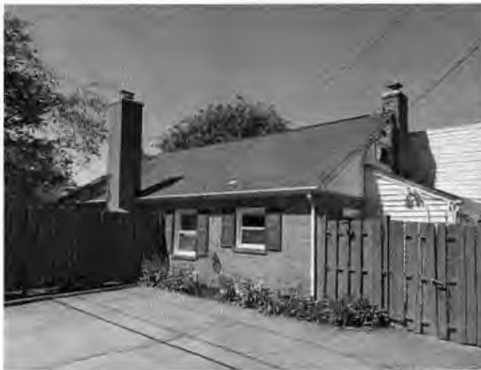
2. 1413 MT. VERNON AVE SIDE AND REAR FACADE
