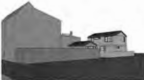
South Facade (rear)
