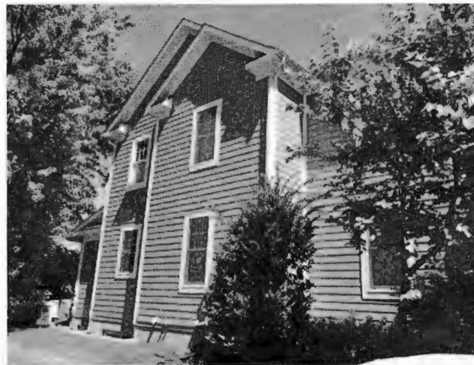
4. 408 E. ALEXANDRIA AVE. WEST SIDE YARD
