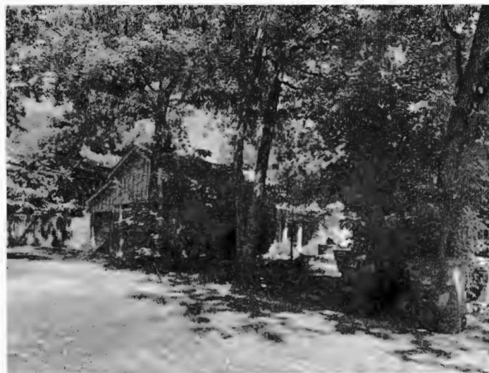
3. 408 E. ALEXANDRIA AVE. DETACHED GARAGE AND ADU
