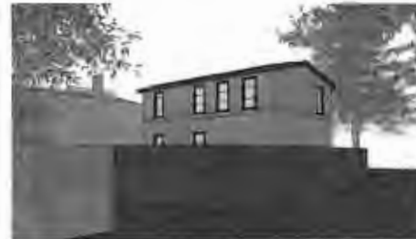
South Facade (rear)
