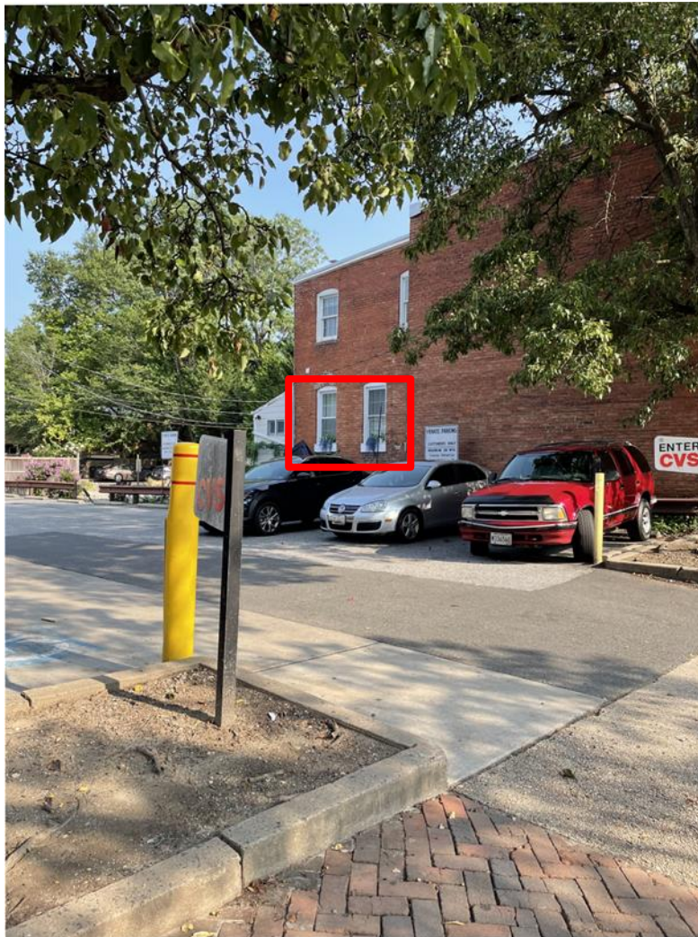
Figure 6 - Windows replaced visible from the ROW.
