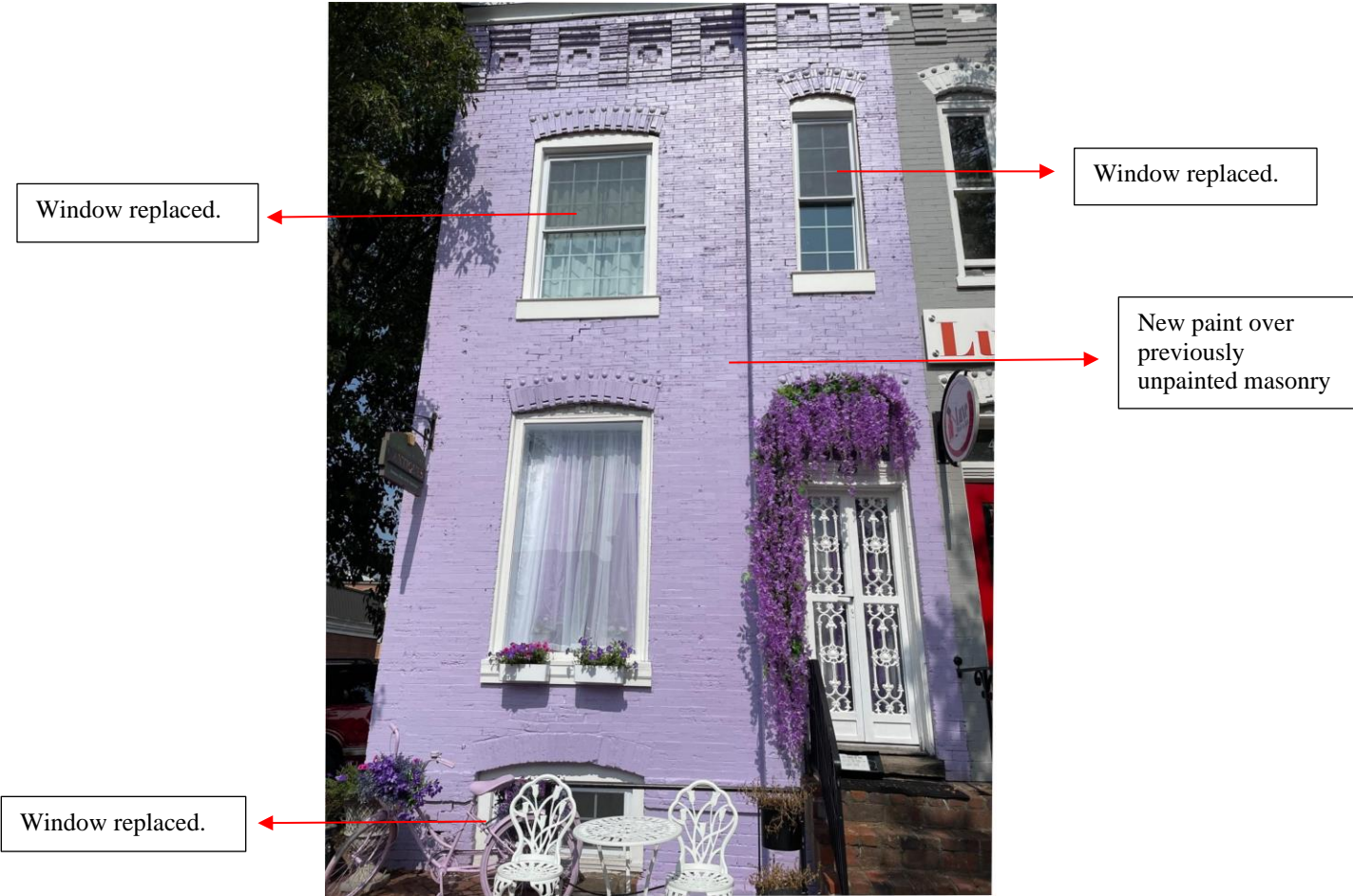
Figure 1 - Painted front/east elevation
