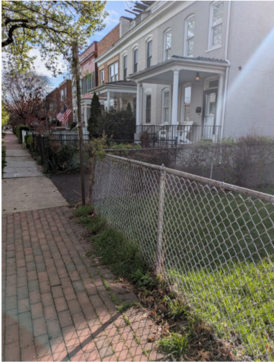
Fence at Corner of Fayette Street and Alley:
