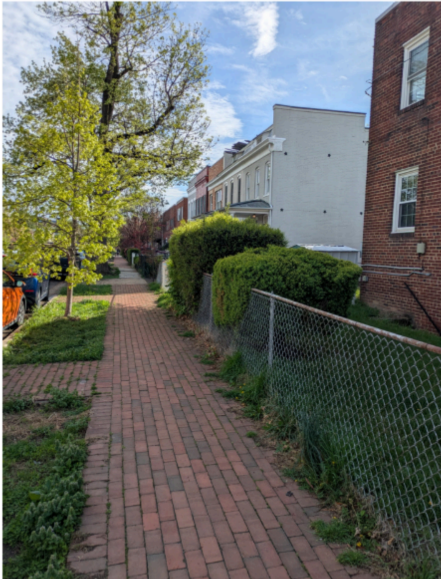
Side Fence on Fayette Street:
