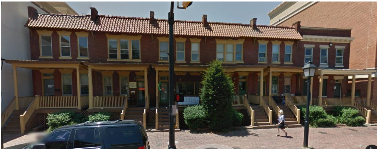
Figure 1: Photo of existing site
