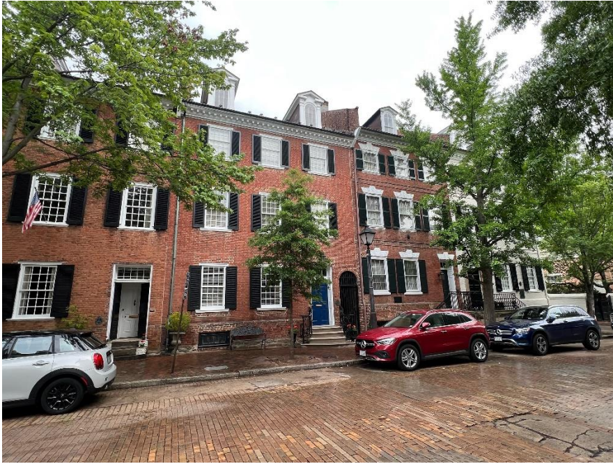
Street view of 211 Prince Street with new handrails on existing steps
