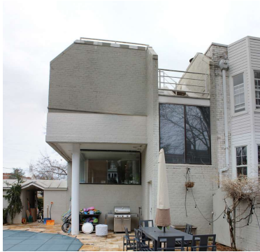
East facade @ Alley
