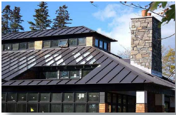
Metal roof examples (standing seam metal @ ±21" o.c.)
