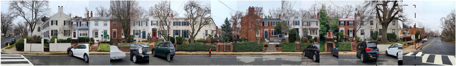
Existing Streetscape @ Royal Street
