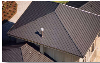
Metal roof examples (standing seam metal @ ±21" o.c.)
