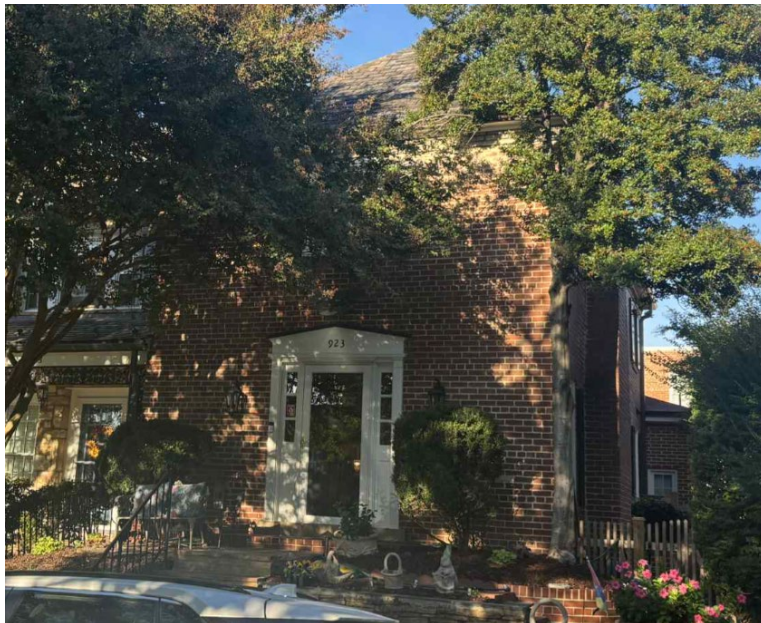
Figure 1. Photo taken by staff of front slate roof, from Saint Asaph Street.
