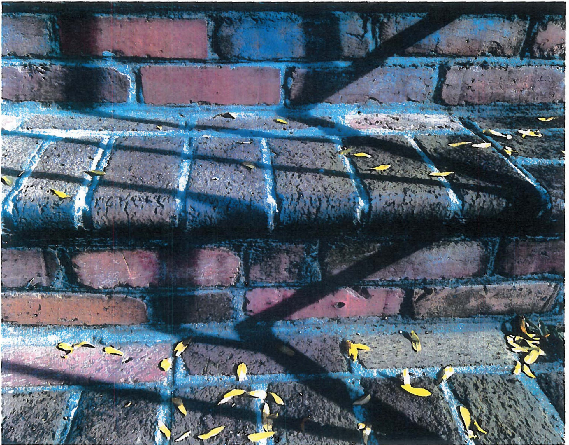
Steps 823 Queen Street – close view of front of steps with
