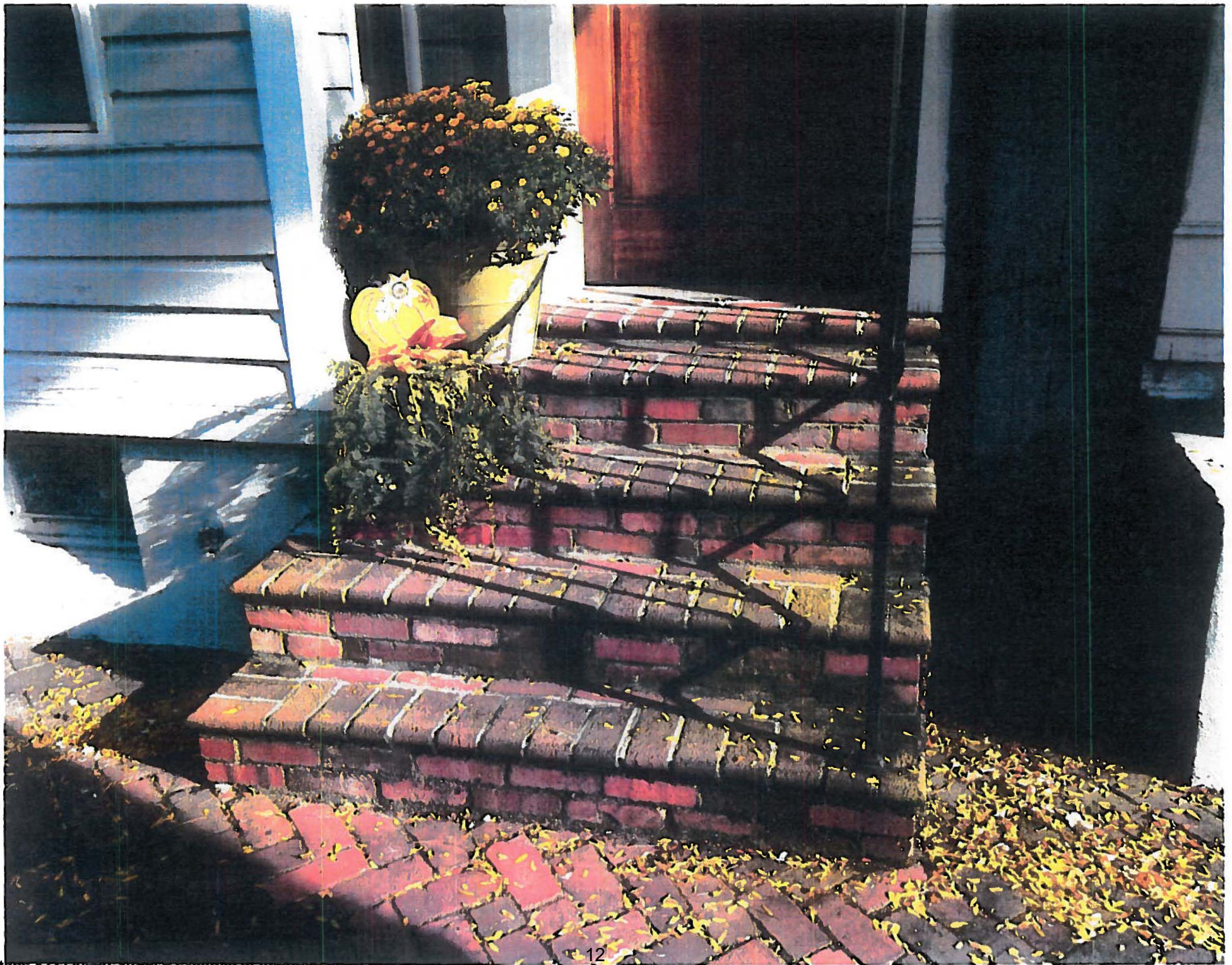
Steps 625 Queen Street - example of masonry and design (with bull nose brick on front and side) with iron
