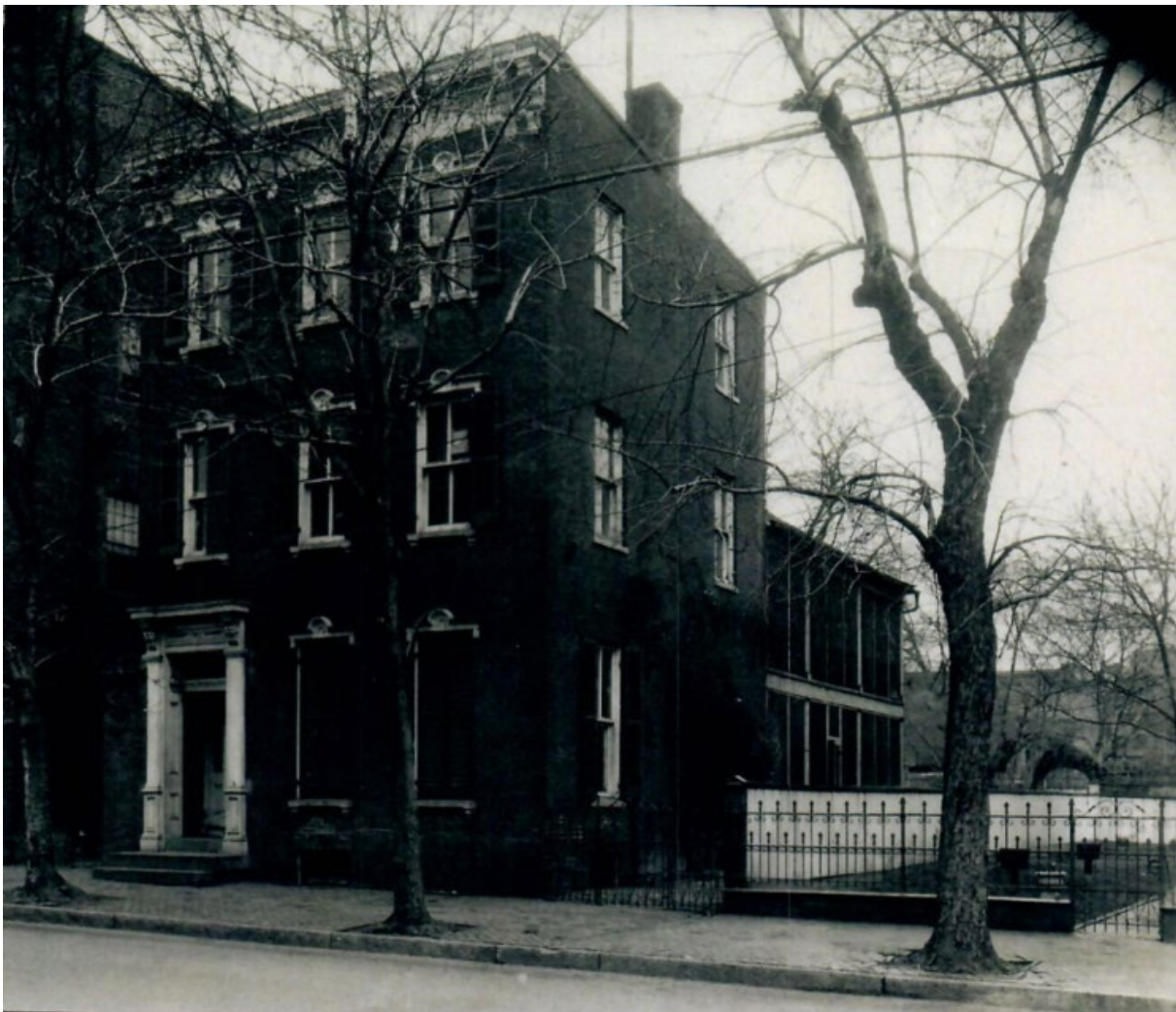
Figure 2: Photograph showing site configuration prior to the construction of the subject brick wall
