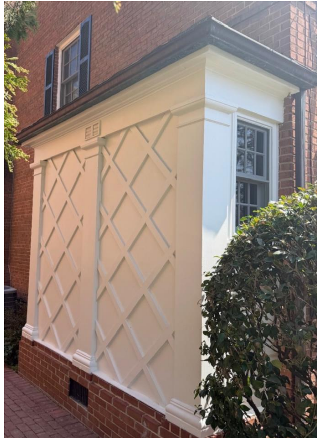
Figure 5: Diamond shaped lattice and pilasters similar to proposed north elevation
