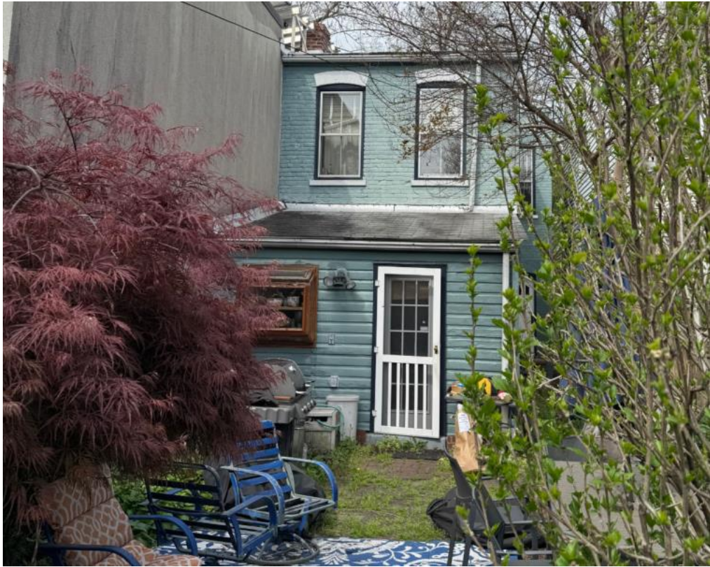
Figure 2: Existing frame one story addition to be demolished
