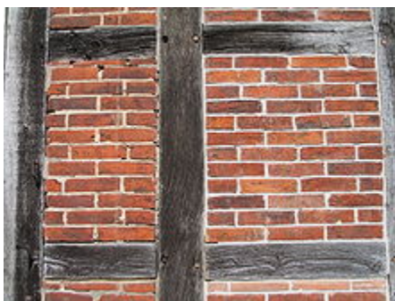
Example of timber framing with brick nogging.
