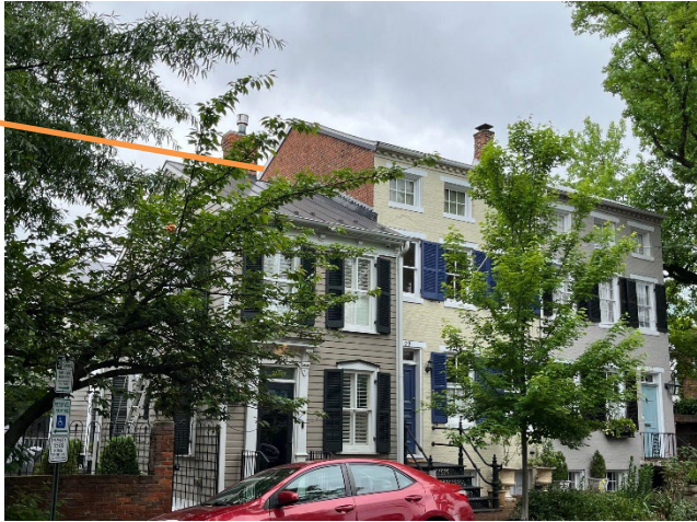
Figure 4: Visibility of the third floor rear roof area from Gibbon Street (west elevation)
