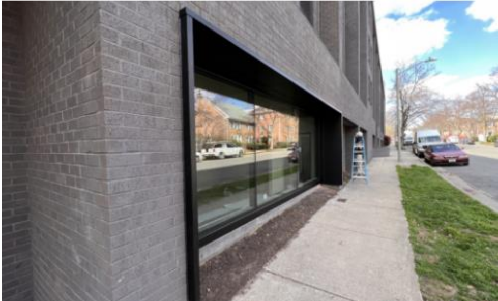
Photo 2: New storefront windows to match existing design on south elevation.
