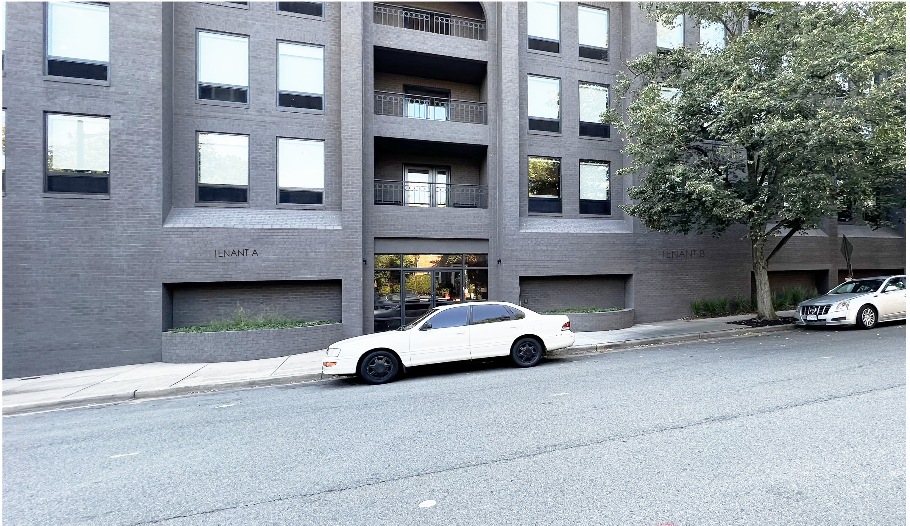
PITT STREET ENTRY EXISTING
