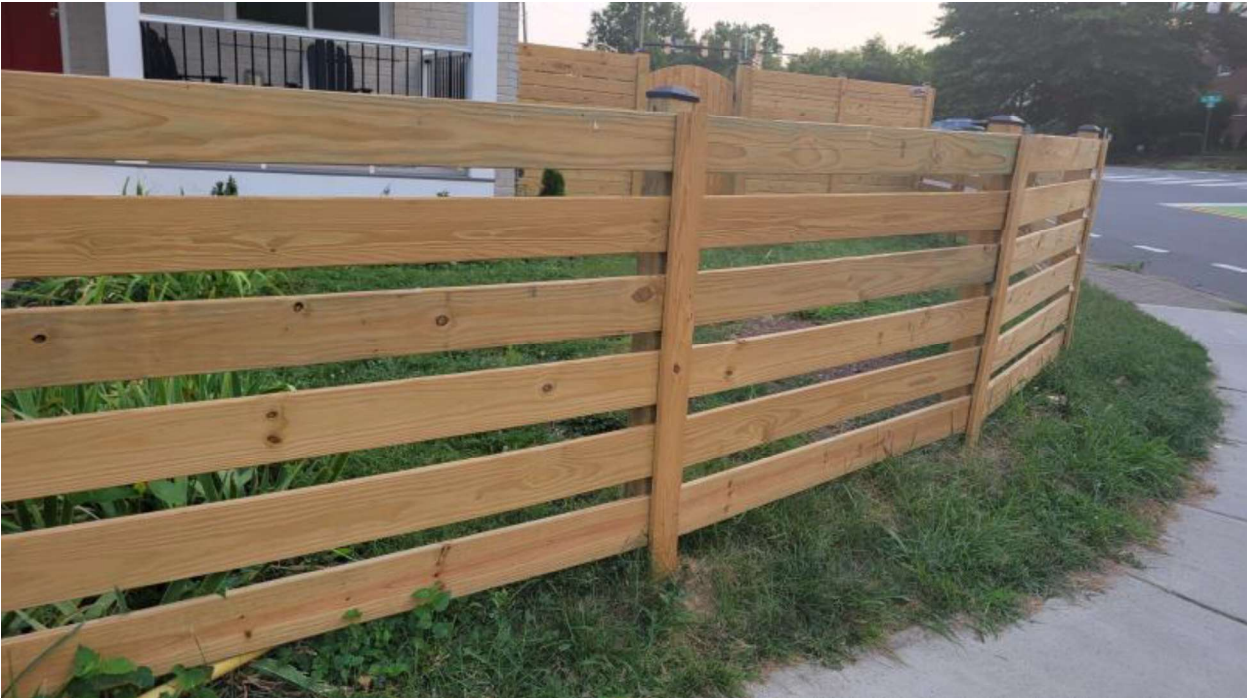
Exhibit 1: Front Yard Fence at 1 Clifford Avenue:
