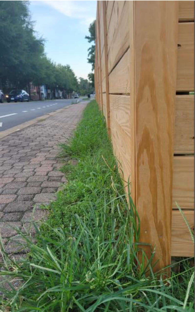
Exhibit 2: Side Yard fence at 1 Clifford Avenue:
