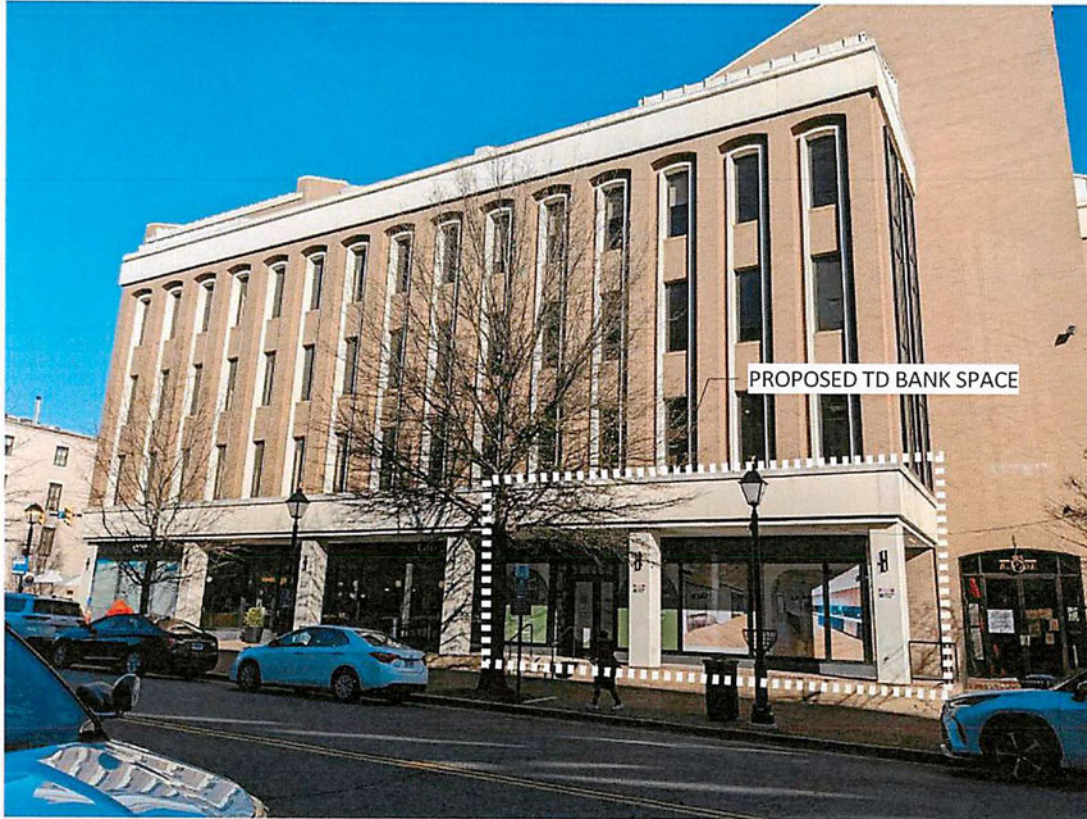
VIEW OF FRONT ELEVATION FROM KING STREET
