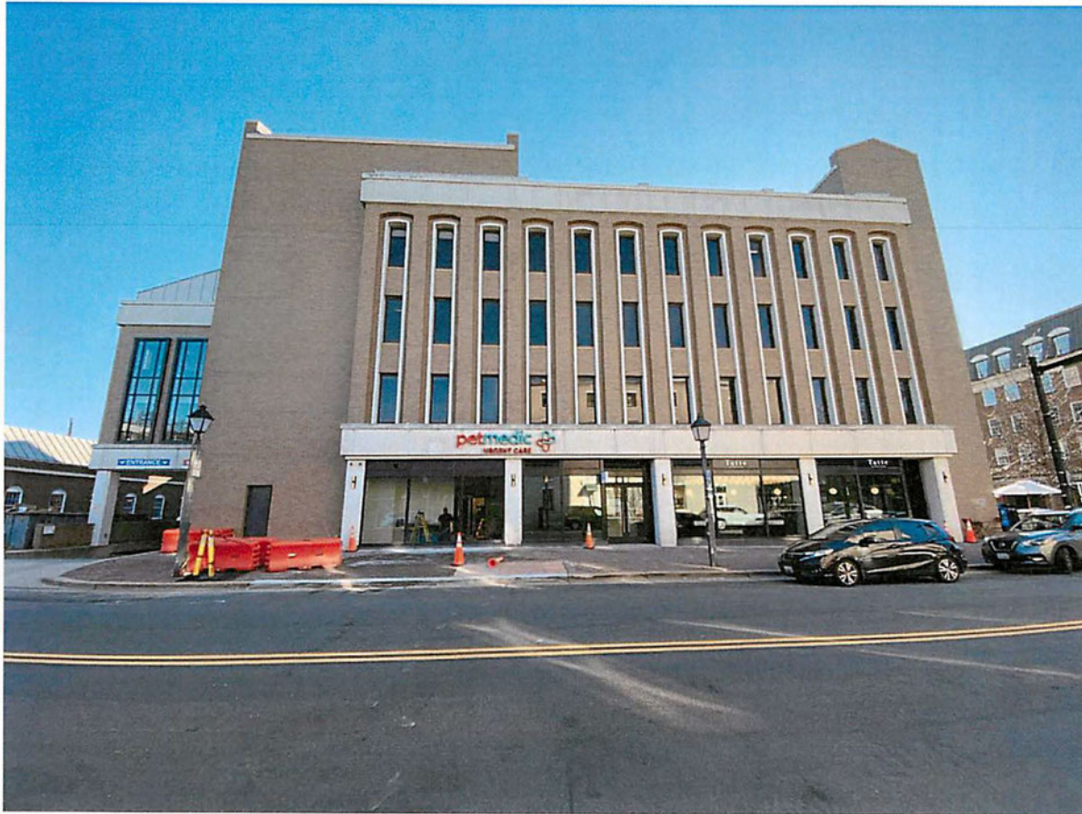
VIEW OF SIDE ELEVATION FROM N. ASAPH STREET
