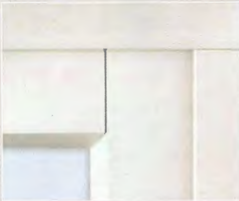
Mortise-and-tenon corner seam with beautiful, clean lines
