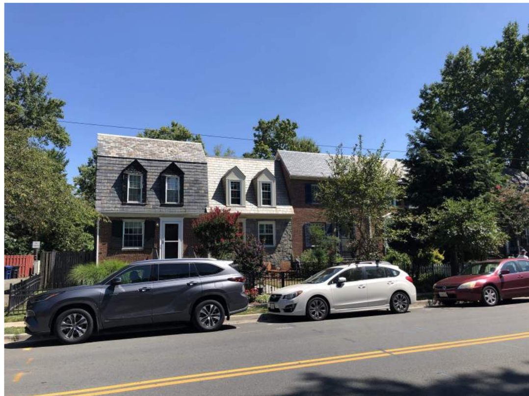
3. 1405 - 1411 MT. VERNON AVE., PUBLIC ALLEY ENTRY ON THE LEFT
