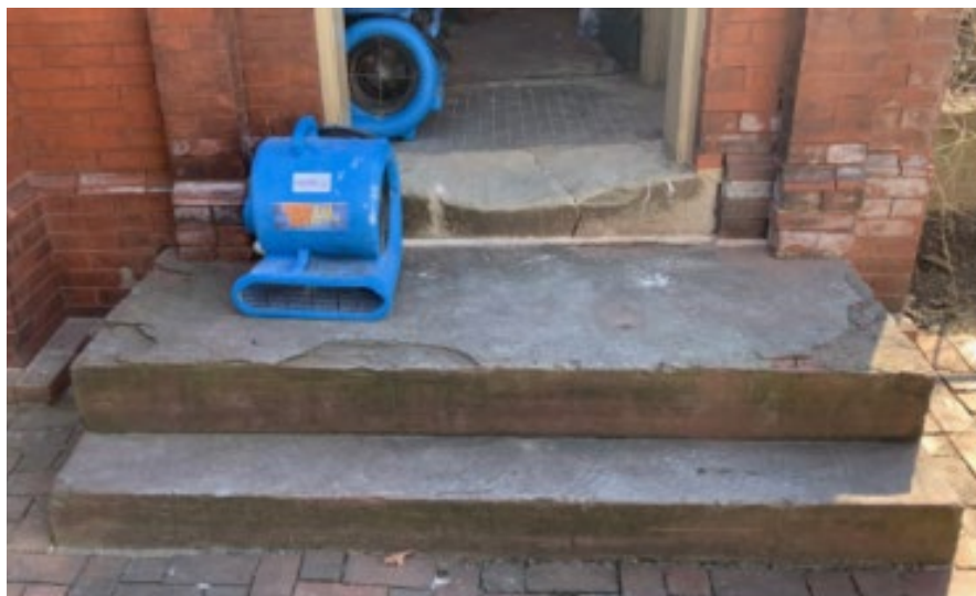
Figure 3: Existing damaged stone threshold block to be replaced in-kind
