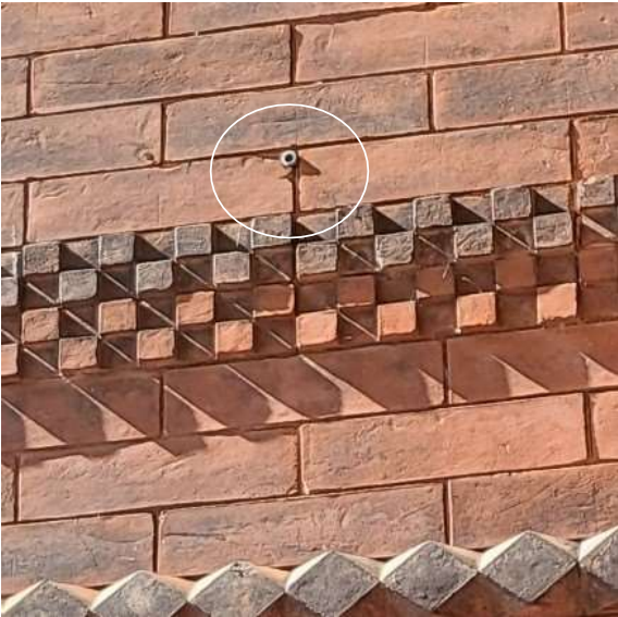
existing anchor location to be used for front security camera wiring
