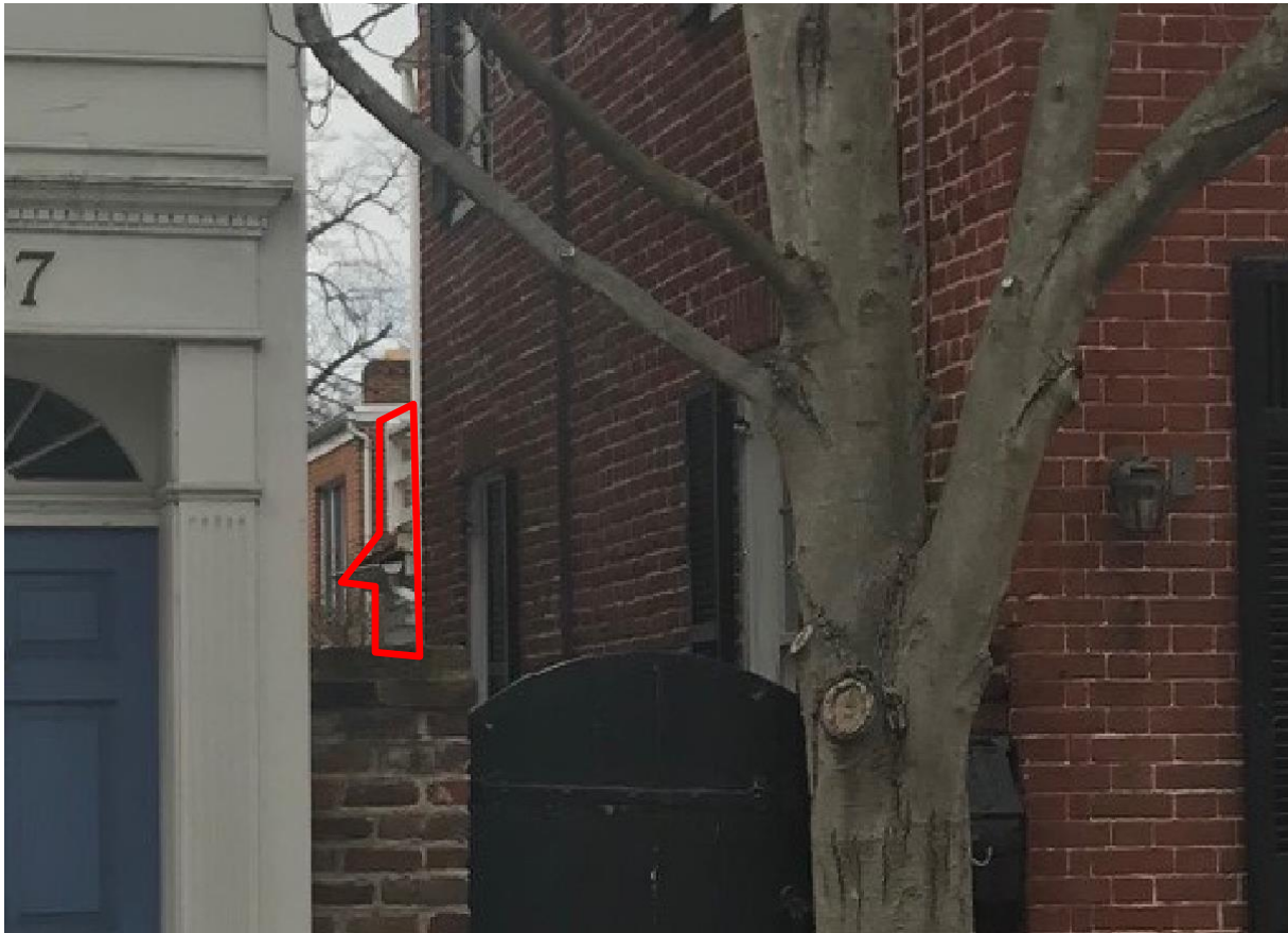
Figure 7: Enlarged photo showing existing visibility of frame ell
