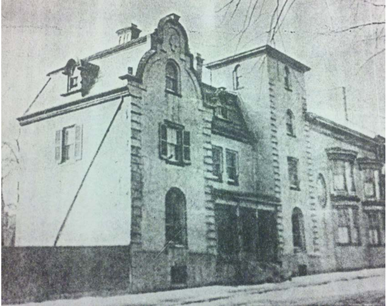
Figure 15. Wolfe Street Townhouse, now Demolished, Showing a Similar Front Gable Form
