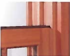
Wood jambs with removable sash stops
