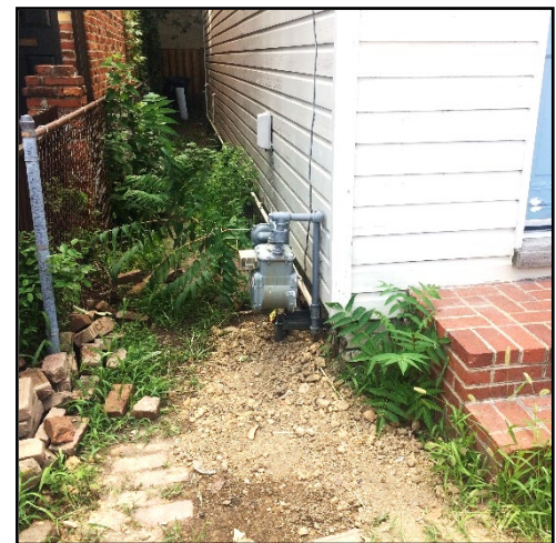
Meter may be located in the side yard behind the façade. Paint meter to match adjacent wall color and screen with landscaping or a fence.
