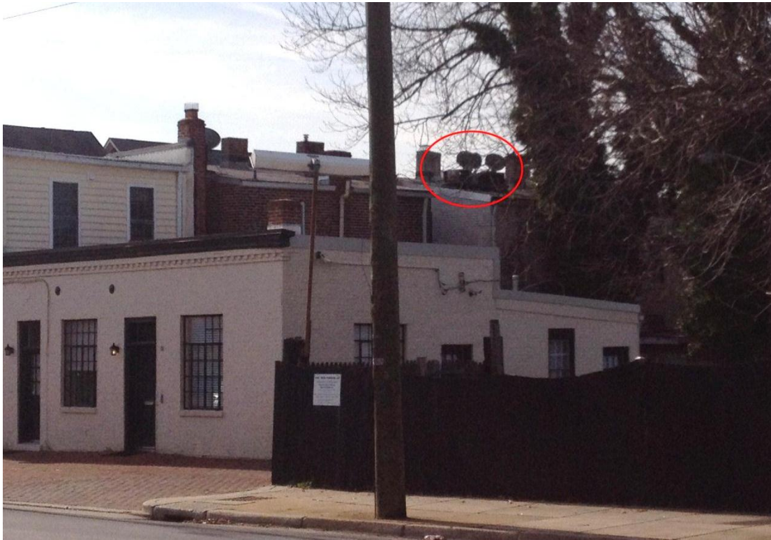
Figure 2: View from South Henry Street showing location of rooftop mechanical equipment.
