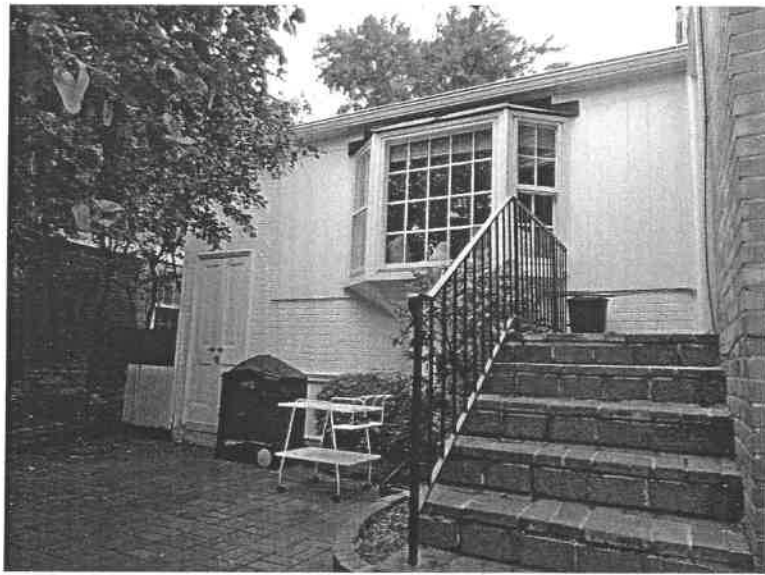
801 S Royal - East View of Existing Addition
