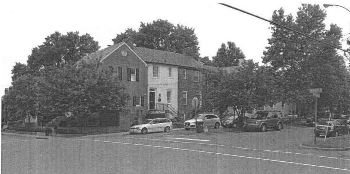
Corner of South Royal / Jefferson Streets - Northeast View
