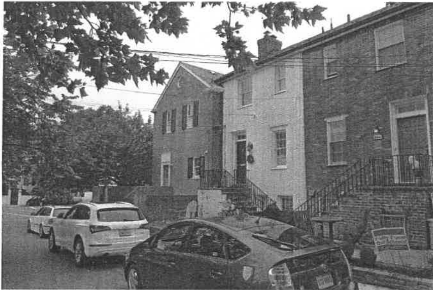
Front- Jefferson Street - Northwest View
