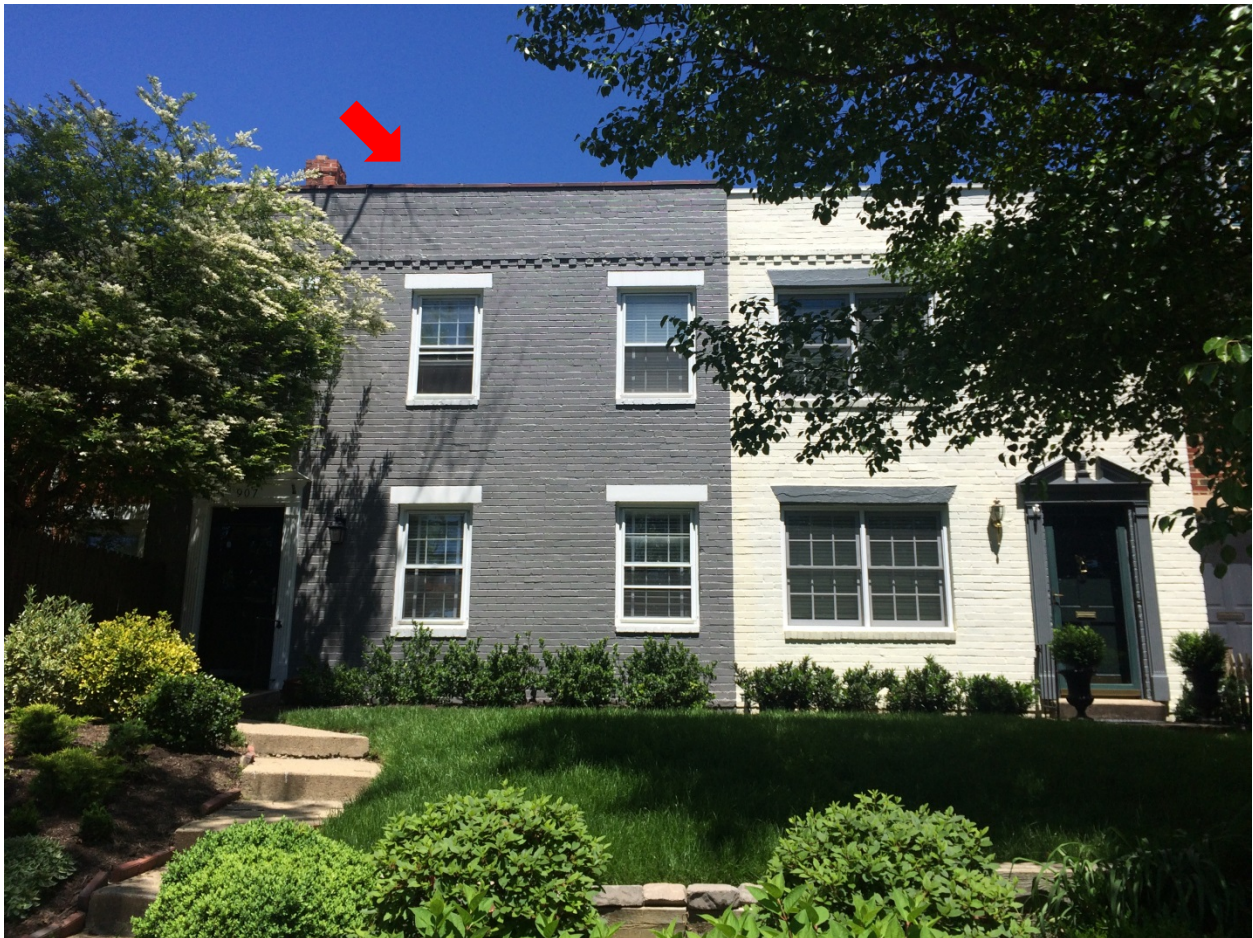
Figure 1: Front (south) façade of 907 Green on the left, painted grey
