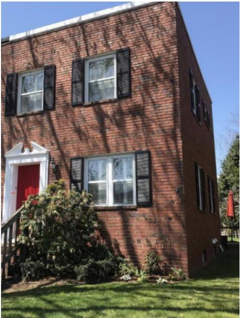
Figure 1: Front elevation of 725 South Alfred Street
