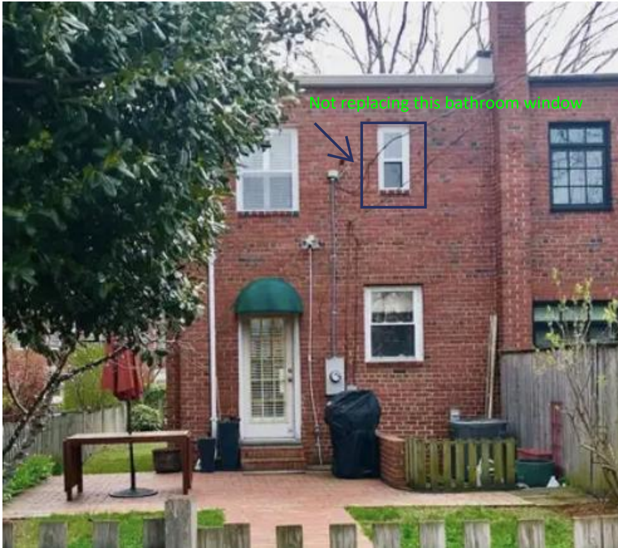
Figure 5 BACK OF HOUSE FAÇADE
