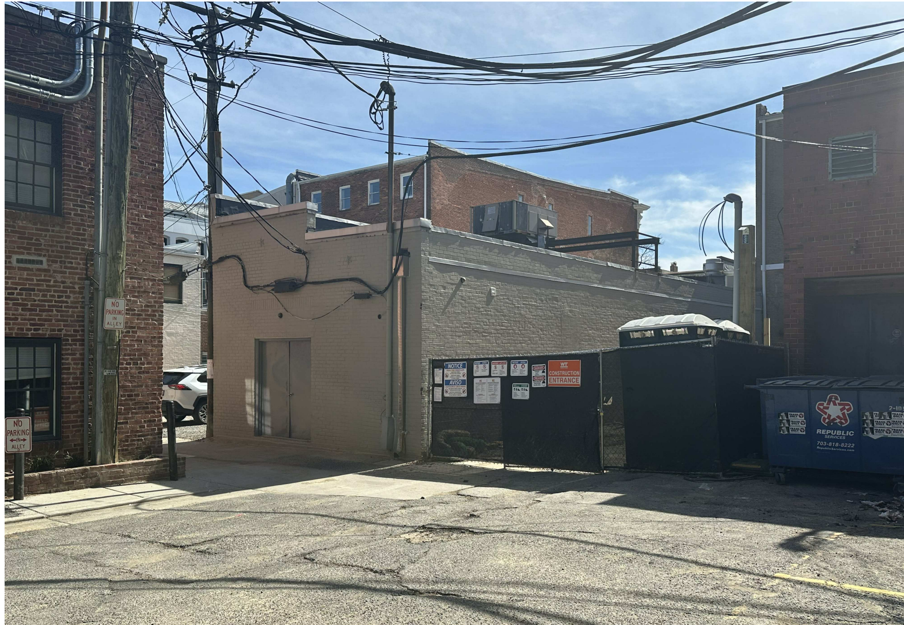
PHOTO AT BACK ALLEY - NW
