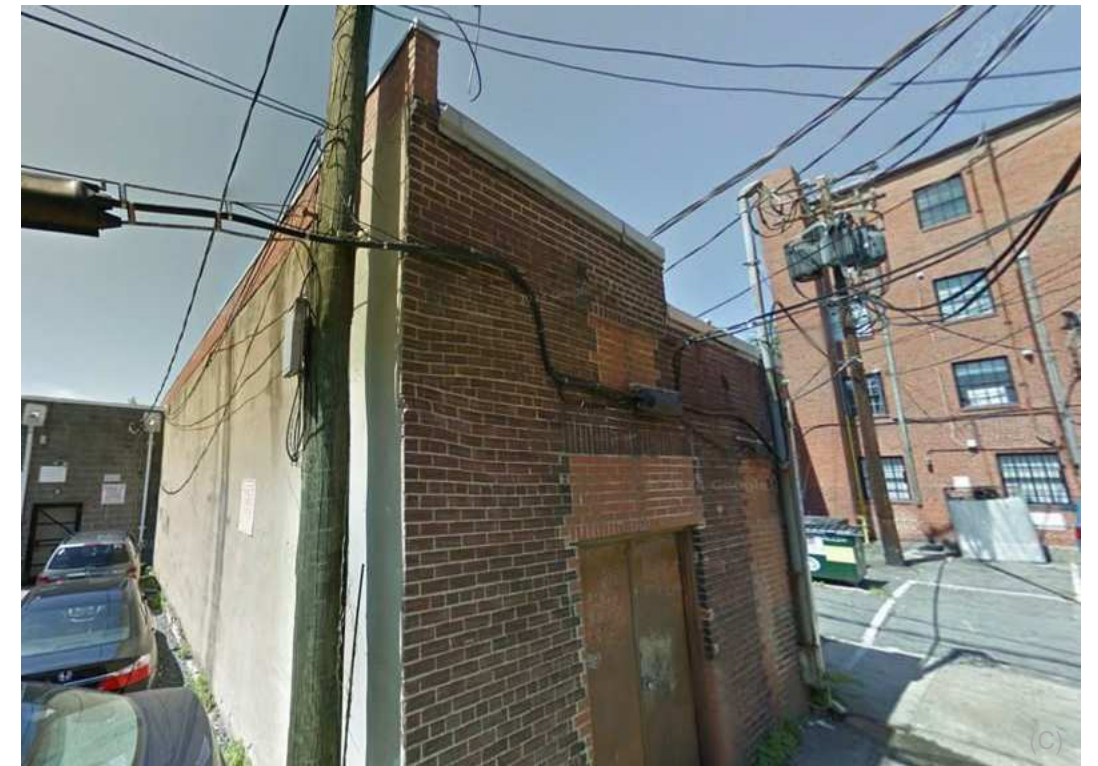
PHOTO AT BACK ALLEY
