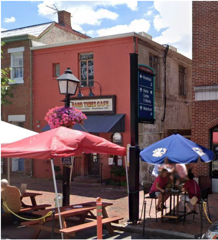
Figure 1: Existing north elevation
