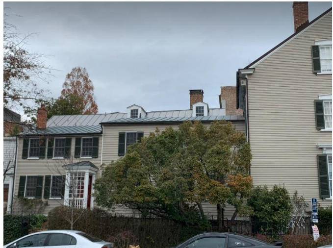
Figure 2 (left). The 1852 massing facing South Saint Asaph Street, with a gable roof. Figure 3 (right). The late 1700s and 1986 massings facing Wolfe Street, with flounder roofs.
