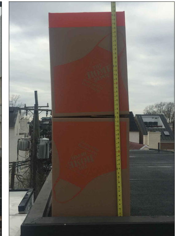
4' TALL BOXES @ CORNER OF NEW ROOF DECK
