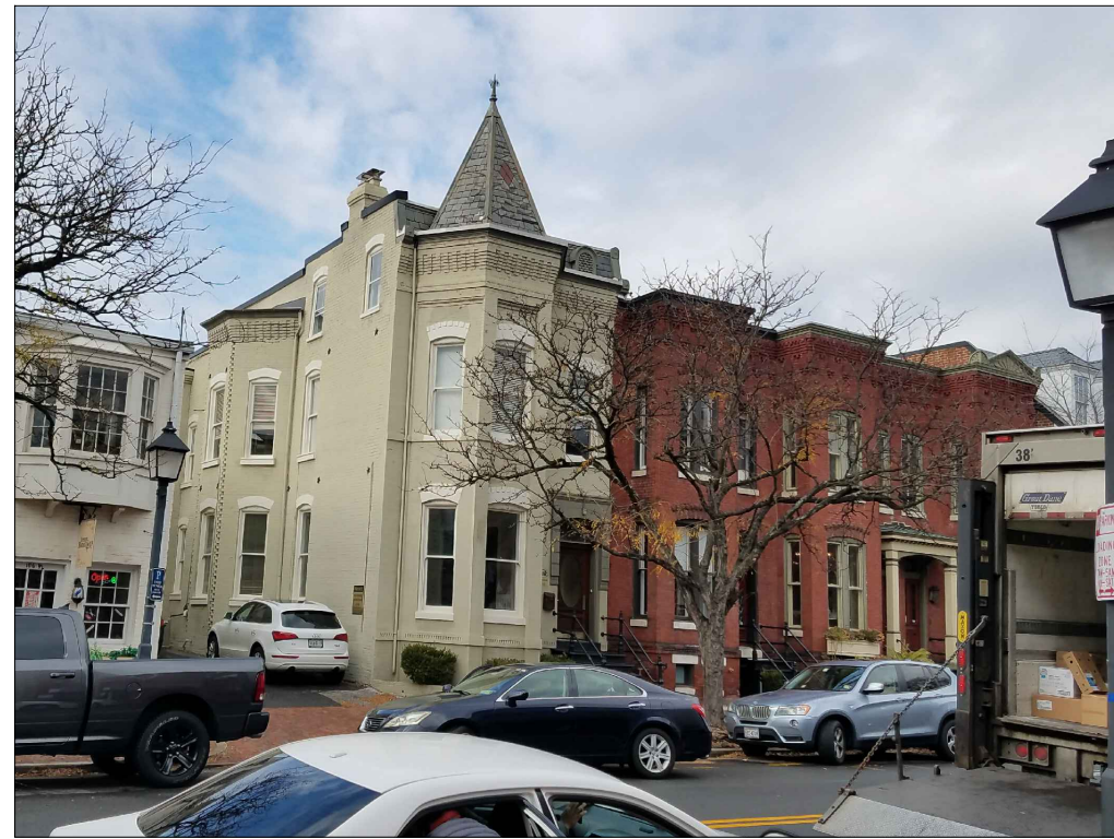
VIEW OF 110 N COLUMBUS ST. FROM THE SOUTH (4' TALL BOXES NOT VISIBLE)
