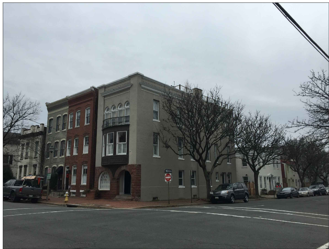
ROOF DECK AT 228 N. COLUMBUS STREET
