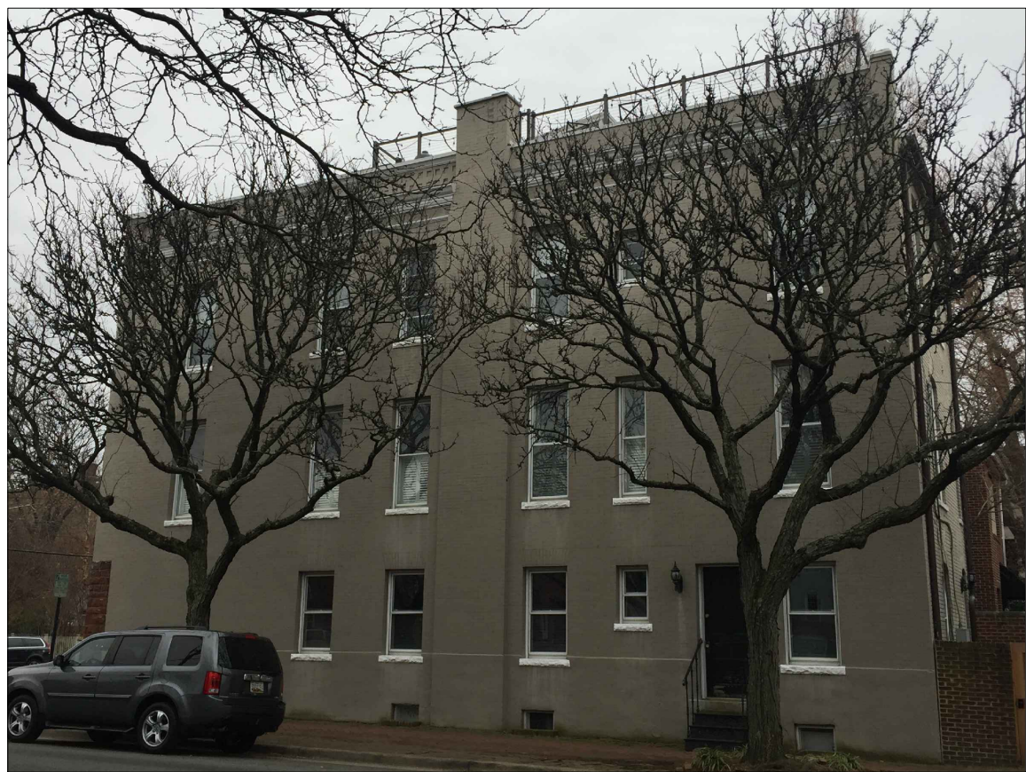
ROOF DECK AT 228 N. COLUMBUS STREET
