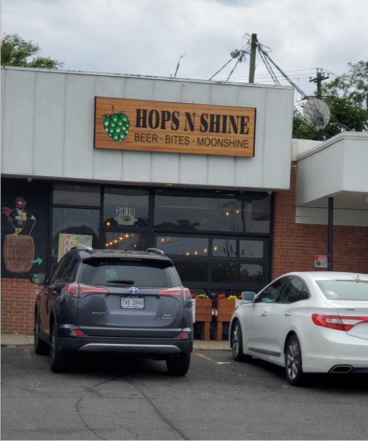
Figure 1 – Building Façade from Mt. Vernon Ave.
