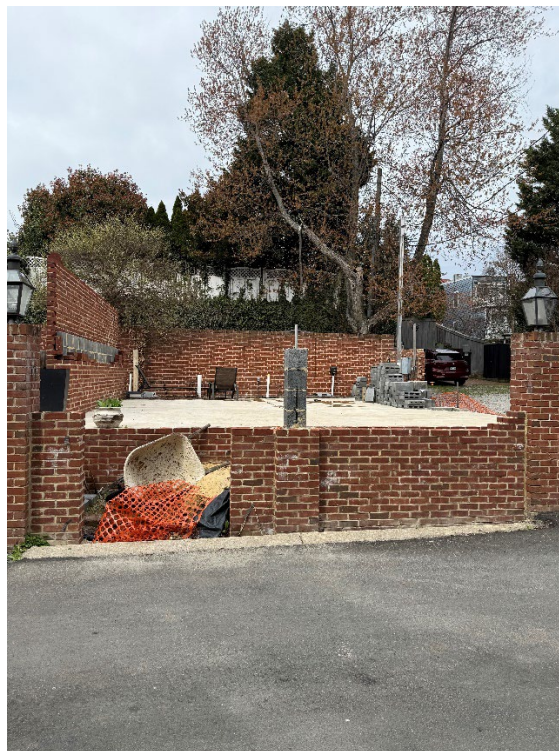
Figure 2 - Garage addition construction today
