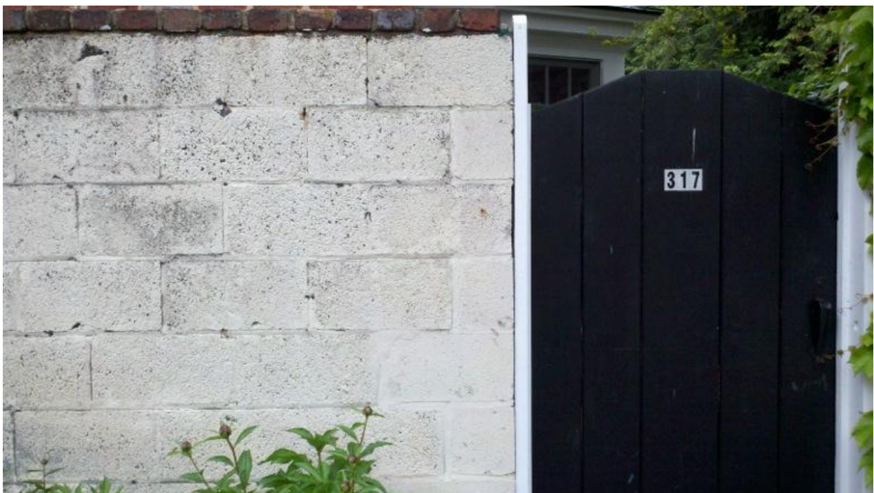
Figure 2: Detail photo of existing cinderblock wall
