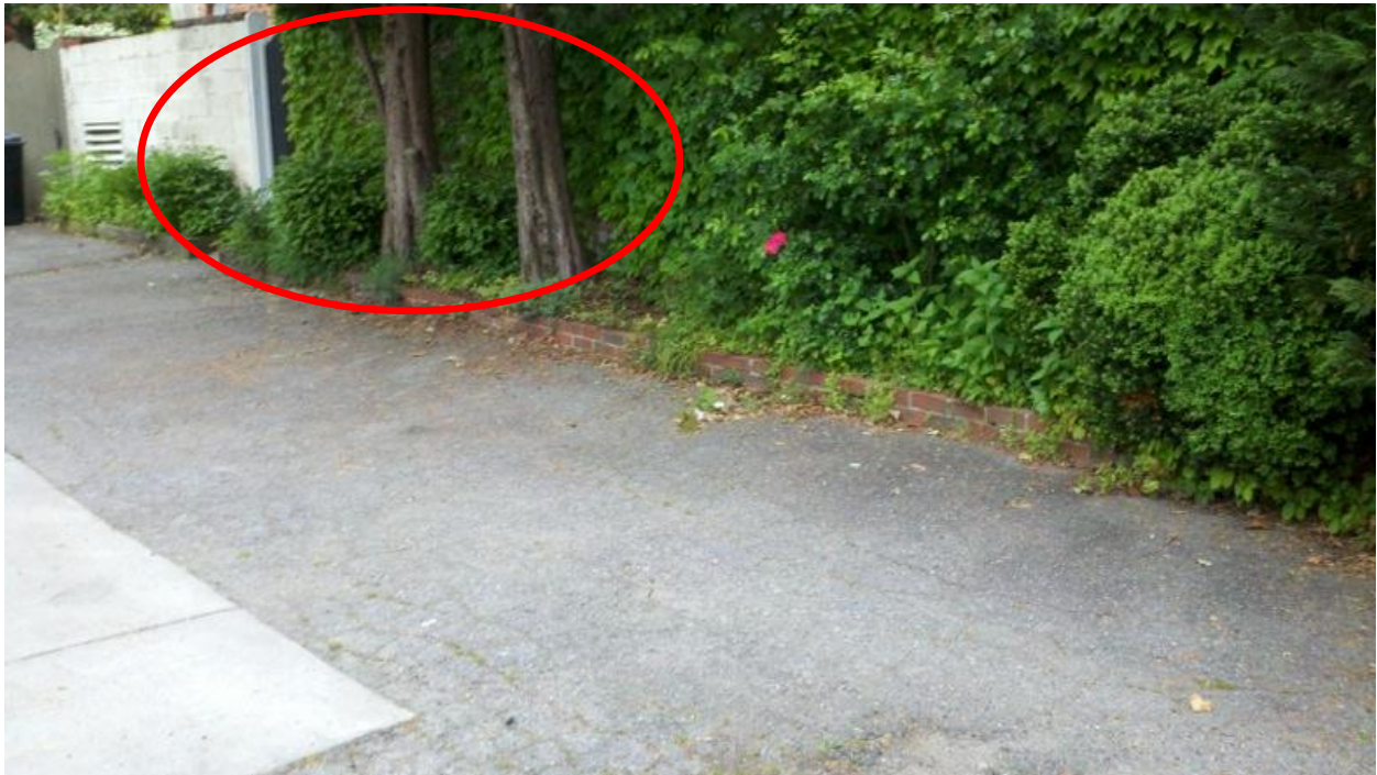
Figure 1: Location of proposed demolition (cinderblock wall is currently covered in vegetation)
