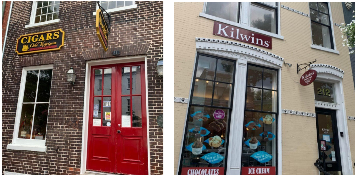
Figure 3: Existing signs at 210 and 212 King Street
