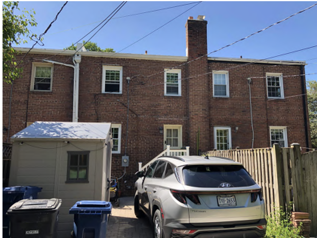
3. REAR FACADES AND YARDS OF 1407 - 1411
