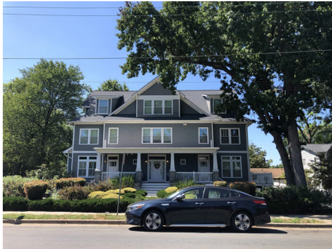
1. NORTHWEST CORNER OF MT. VERNON AVE. & E. ALEXANDRIA AVE.
